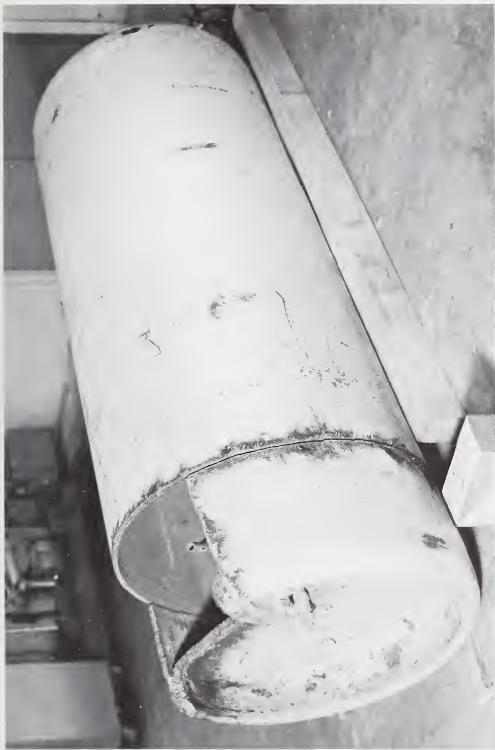
Figure 1. The tank after flame cutting to remove the end that leaked and the section that contained the leak.
