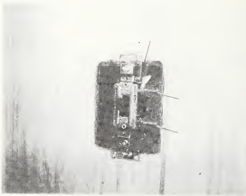
Figure C-100 - Loose Connections (Copper Wire) in Wall Switch
