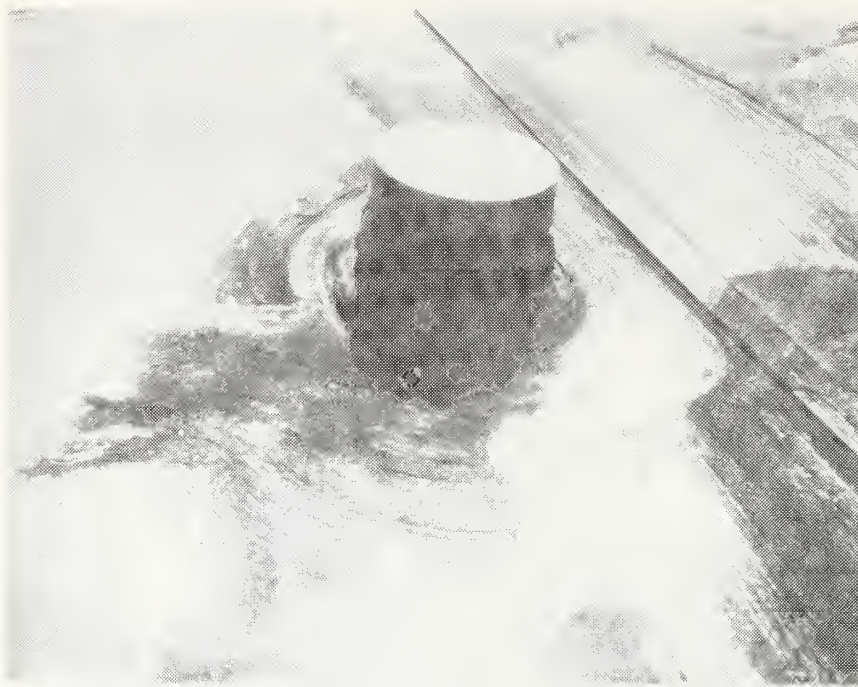
Figure C-76 Vent Cap on Roof Which is Not the Removable Type Required by ANSI A119.1 Standard
