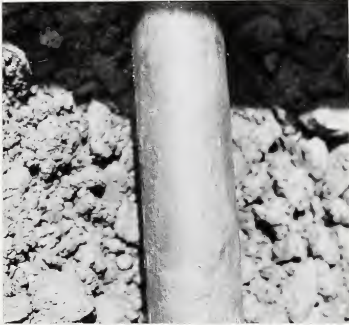
Figure 6. Top view of part of the pipeline excavated at site 2. X ~ 1/2
