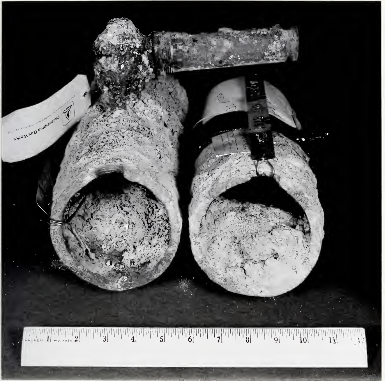
Figure 2. Opposing fracture surfaces as received. The north fracture surface is at the left and the south fracture surface is at the right. Large deposits of soil can be seen inside the pieces of pipe, along with some soil on the fracture surfaces and what appears to be soil adhering to the outside of the pipe. The top of the pipe as installed in the soil is at the top in the photograph. X 1/2
