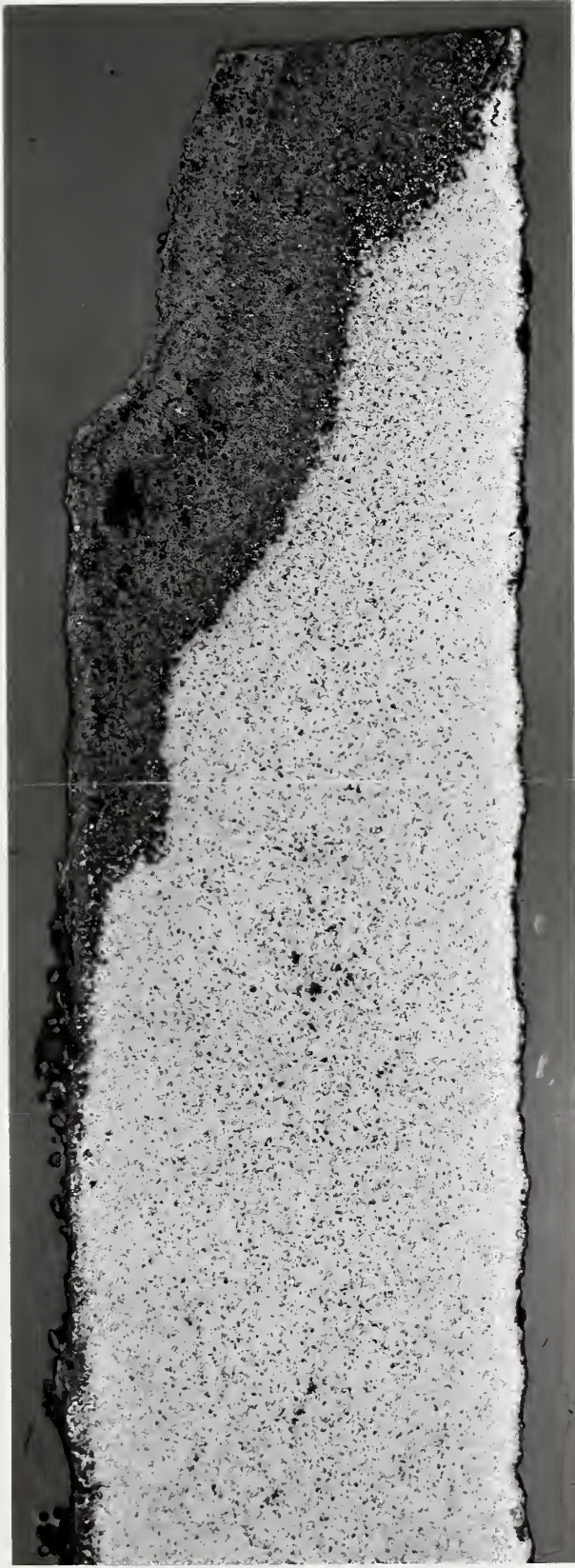
Figure 13. Longitudinal section through the top of the pipe. Right side of the section is two inches north of the fracture. The dark area represents graphitic corrosion, which has penetrated nearly the entire wall thickness of the pipe at the right of the section. Etchant: 1% nital. X 7 1/2
