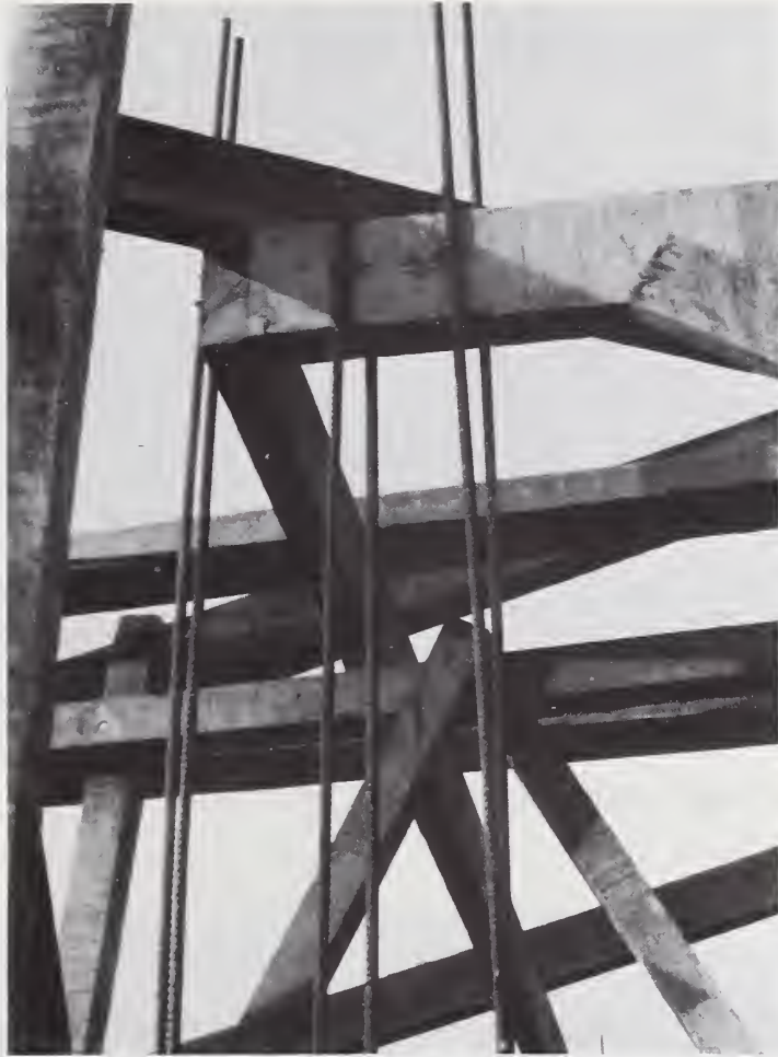
Figure 17 Column reinforcement anchorage to roof rafters
