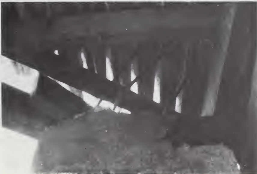
Figure 18 Completed column and roof anchorage
