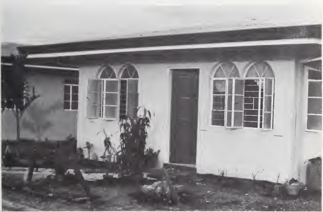
Figure 22 Exterior appearance of completed structure
