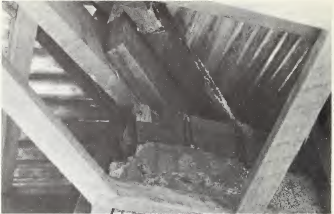
Figure 19 Roof anchorage detail
