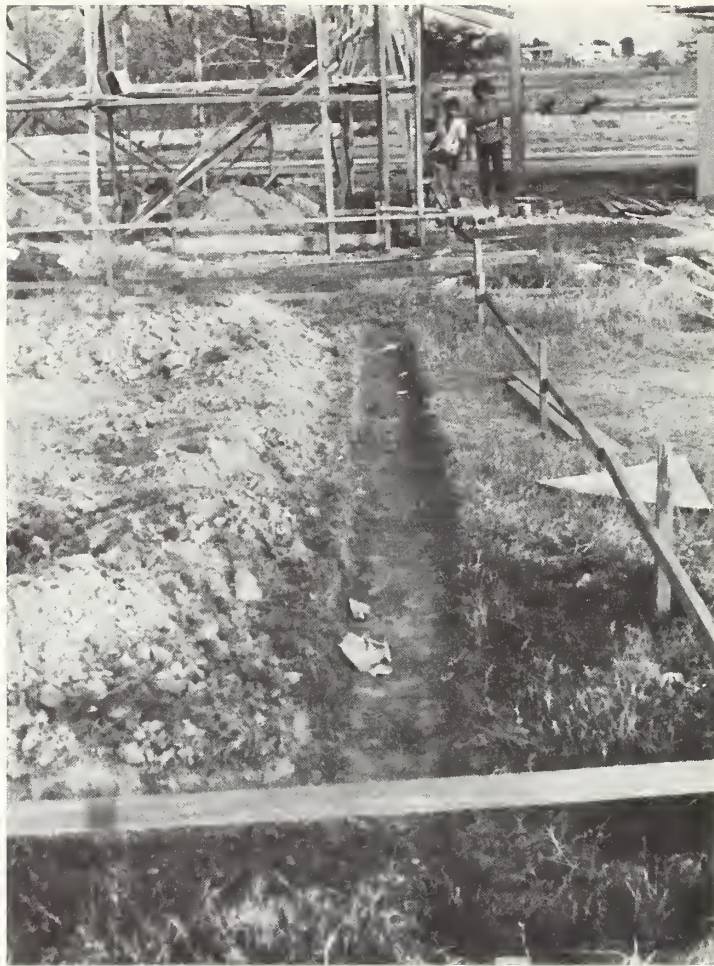
Figure 13 Shallow trench for wall placement
