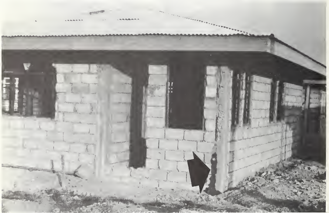
Figure 20 Detail of corner column and exterior wall
