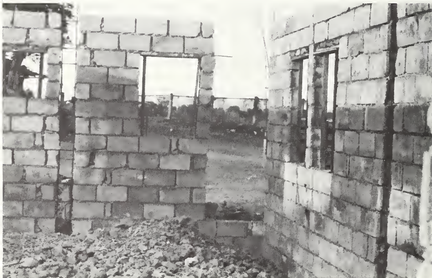
Figure 14 Wall construction quality and window framing details
