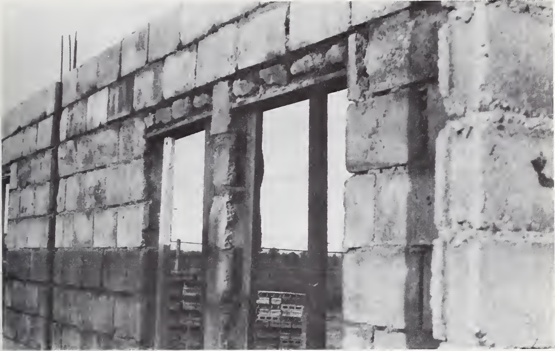
Figure 21 Window framing detail
