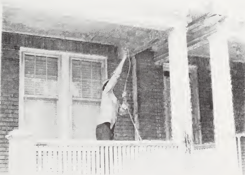
Figure 4. Application of paint remover on painted wood surfaces with spray equipment.
