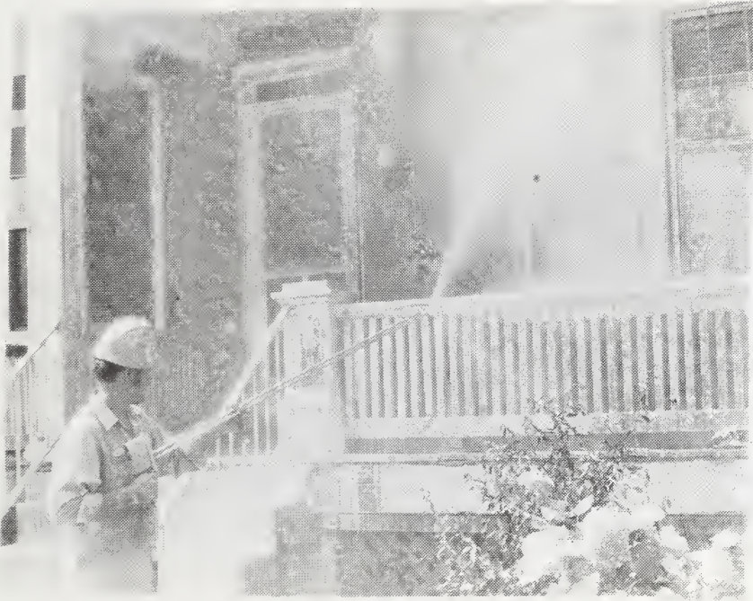
Figure 9. Flushing off old paint with high pressure water spray after treatment with paint remover.
