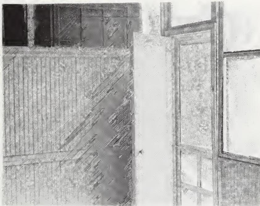
Figure 17. Interior view of wall and door of screened porch after removal of old paint and repainting.
