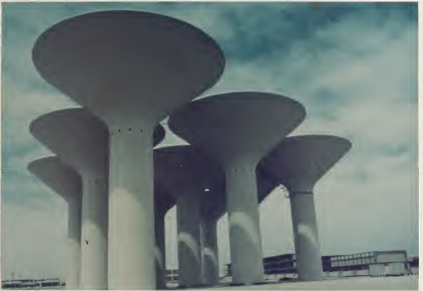
Figure 3. Towers site D-1. Stainless steel type 304L pipes perforated at time of inspection in April 1973.
