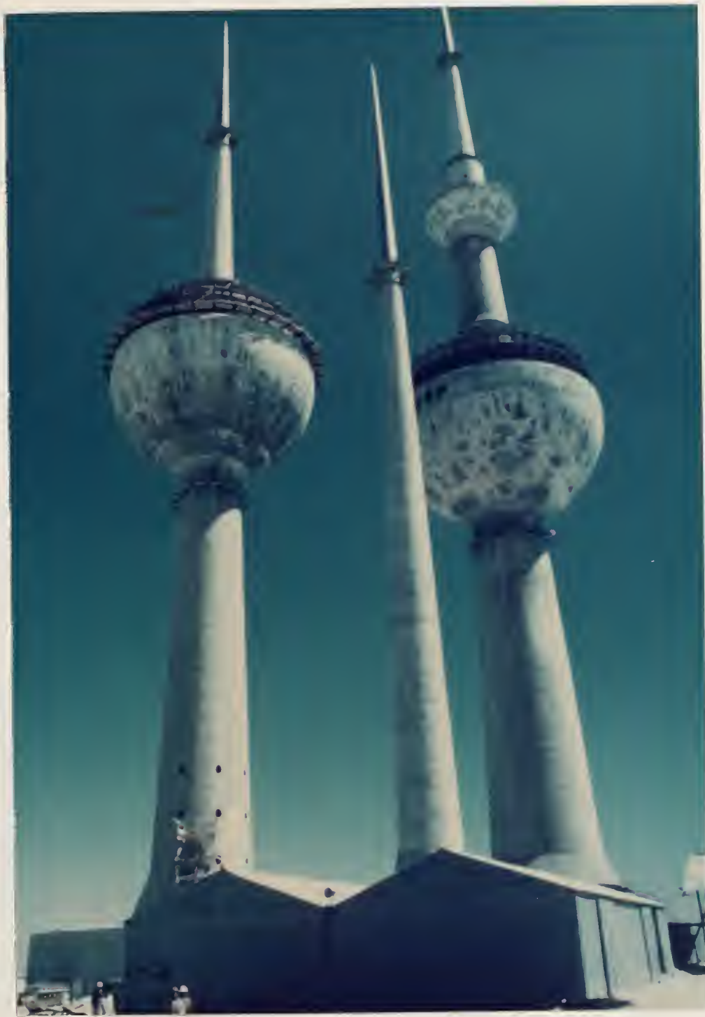
Figure 2. Kuwait Towers, site D-6, water storage towers, and visitors' center as of April 1973. Stainless steel type 316 pipes installed and protected externally with polyethylene.
