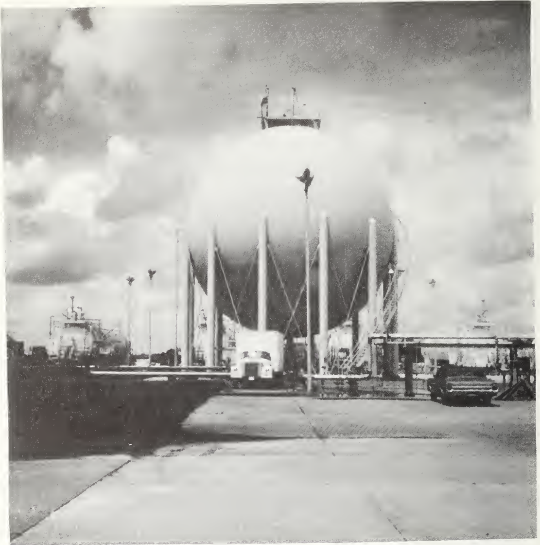
Figure 1. LOX storage tank.
