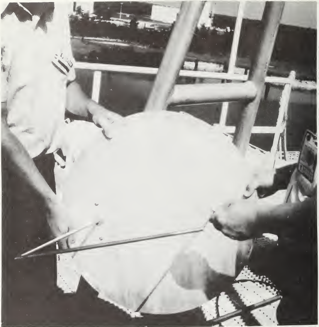
Figure 5. RF loop antenna.
