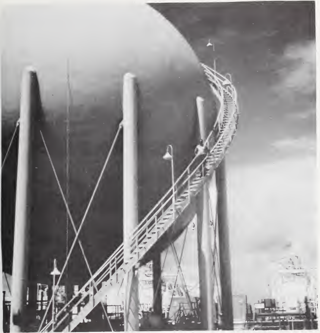
Figure 2. LOX tank stair access.
