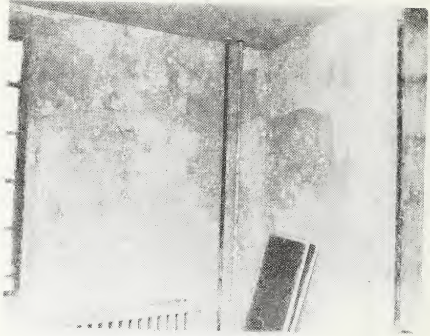
Figure 6. Metal window frame and section of left steam pipe after removal of paint before buffing with steel wool.
