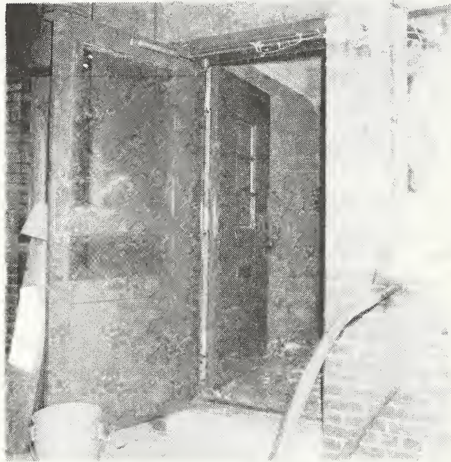
Figure 11. Re-finished wood exterior door, screen door and frame.
