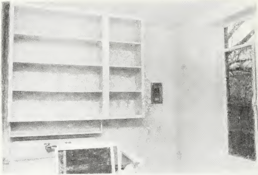
Figure 10. Re-finished plaster walls, shelving and metal window in kitchen.
