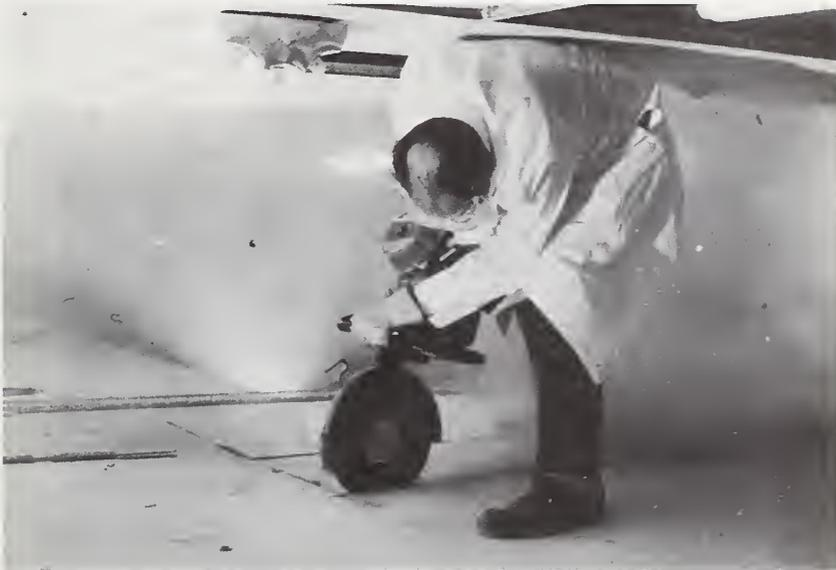
Figure 43. Abrasive Wheel Cutoff Saw
