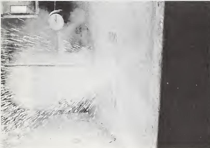
Figure 73. Burning Bar Melting a Hole through Concrete
