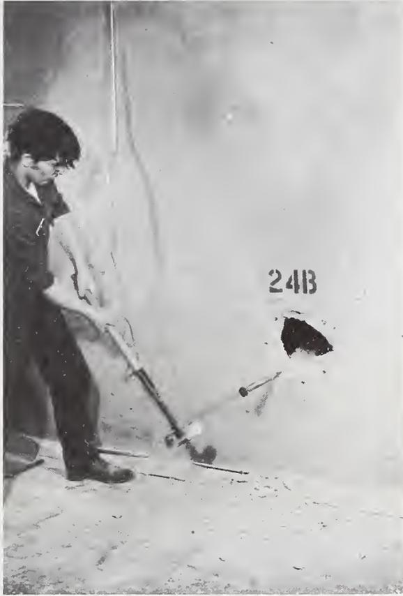
Figure 64. Use of Tapered Punch
