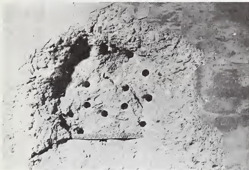
Figure 55. Interior of the Wall with Spalling Nearly Complete
