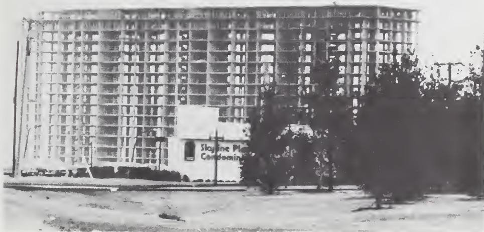
Figure 2.36 Appearance of construction in early February, looking south.
