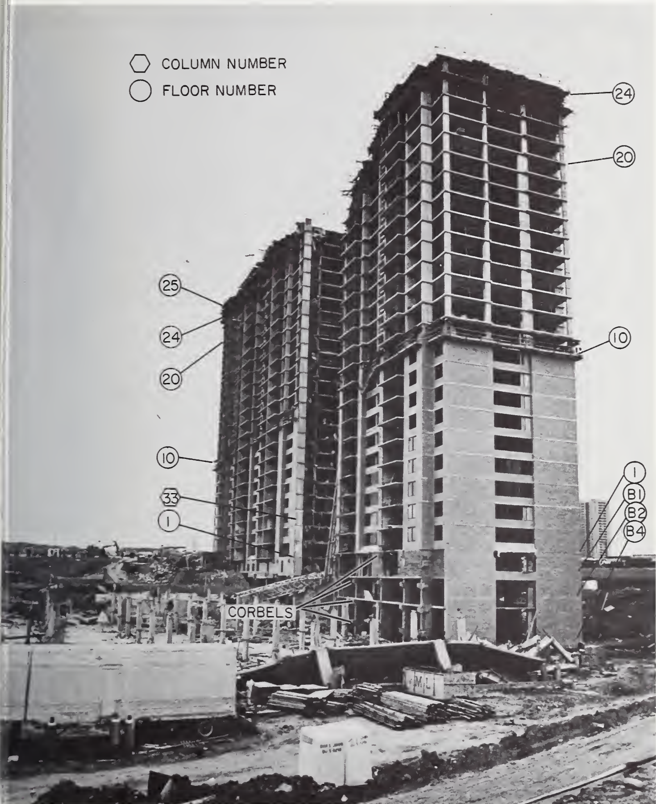
Figure 2.4 General appearance of building A-4 as viewed from the southeast.
