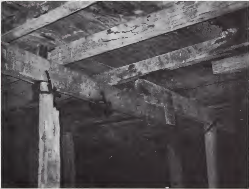
Figure 2.22 Selected details of 23rd story forms.
