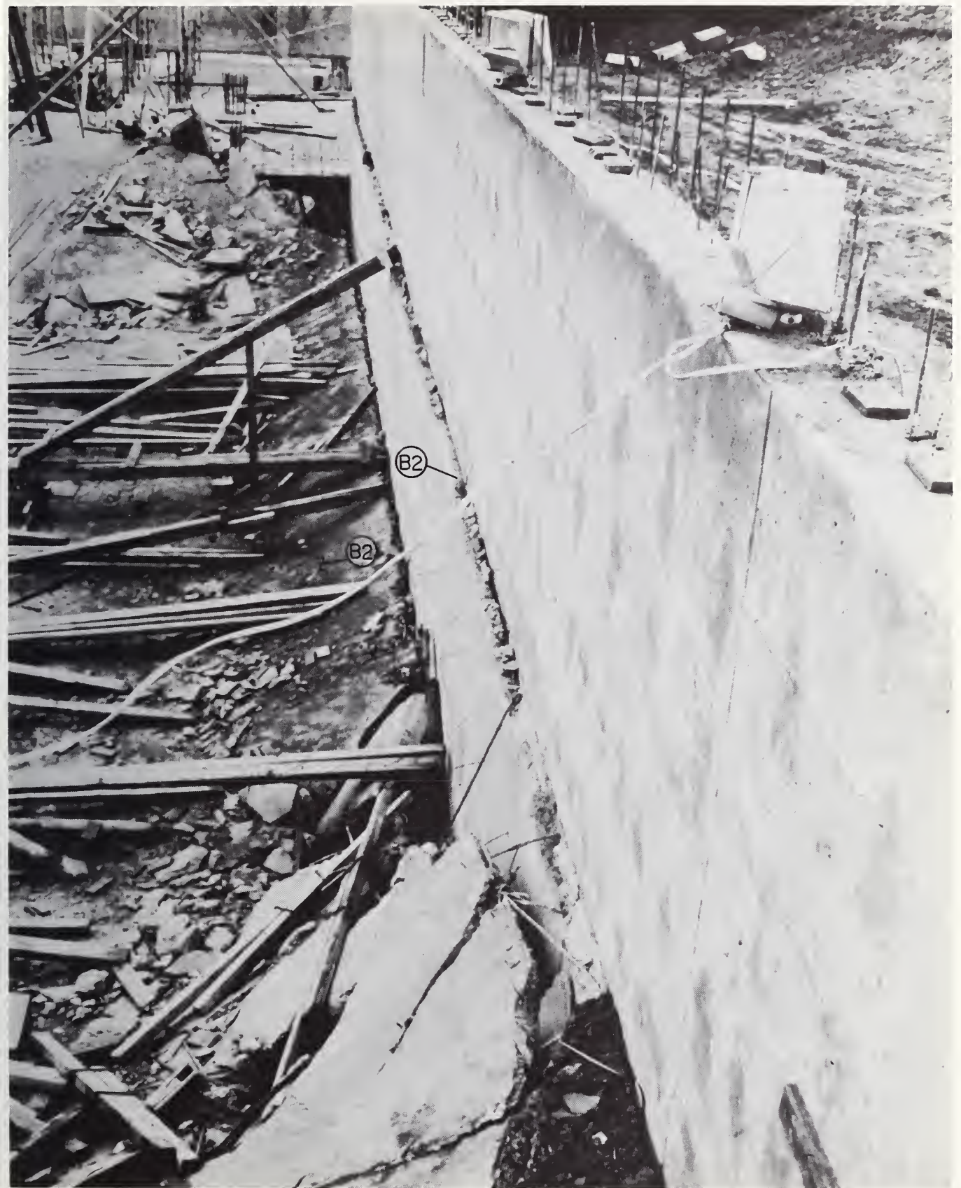
Figure 2.54 Slab support on western wall of parking garage.
