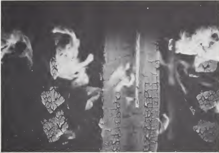
Figure 9. Note the corner reinforcement separating from the column. Test time of 12 minutes.
