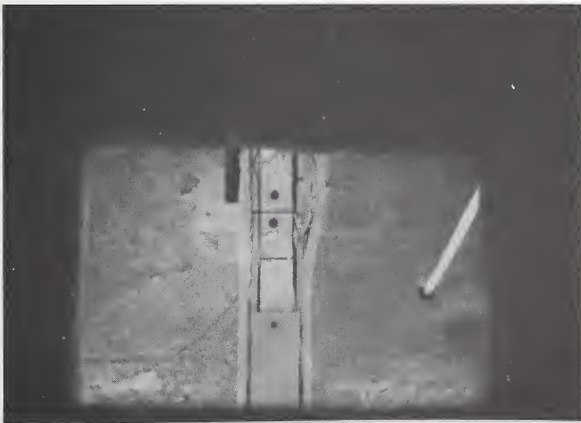
Figure 10. Gypsum covers on the column are falling down. Test time of 45 minutes.
