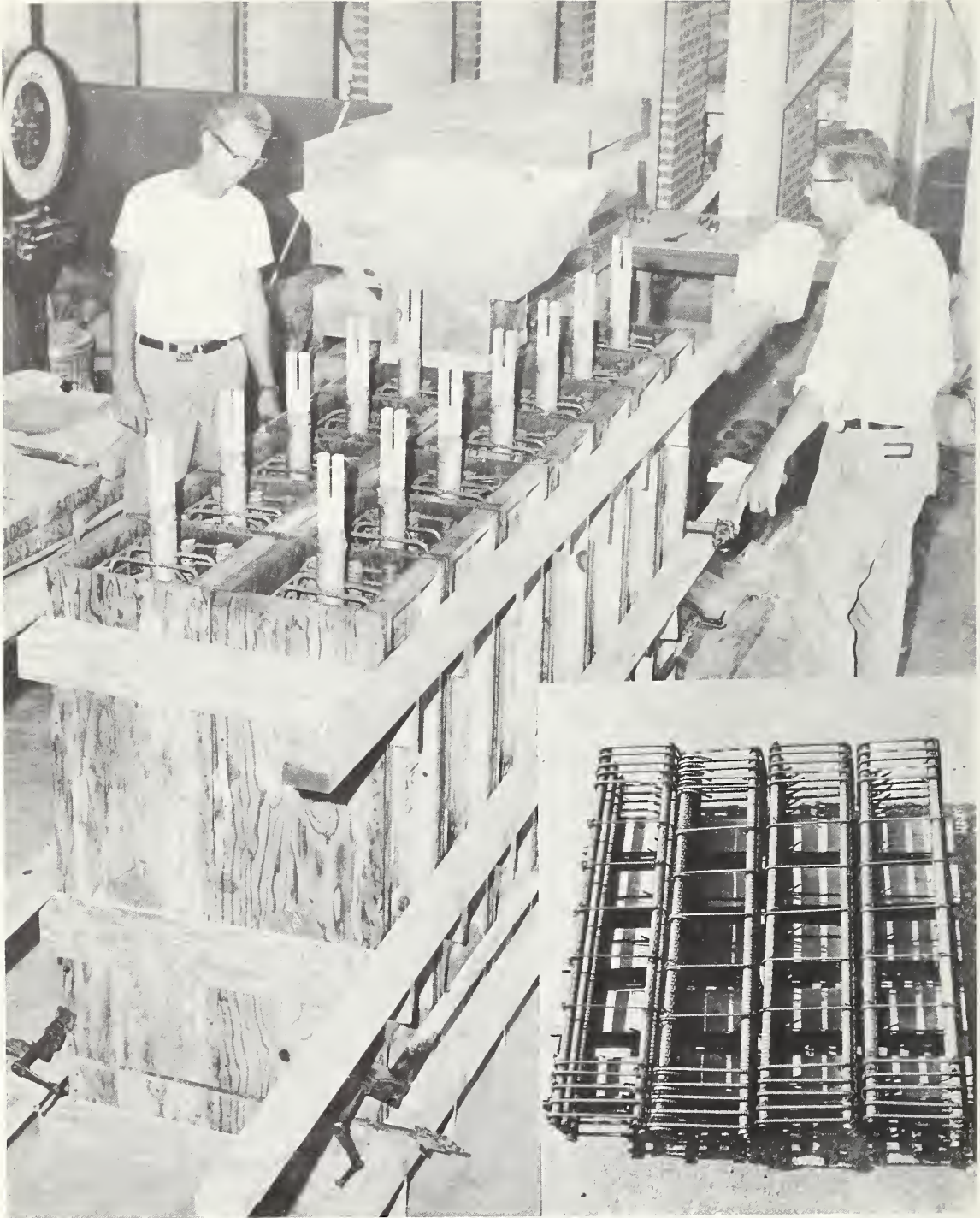
FIGURE 4.20 DETAILS OF SHEAR TEST SPECIMENS
