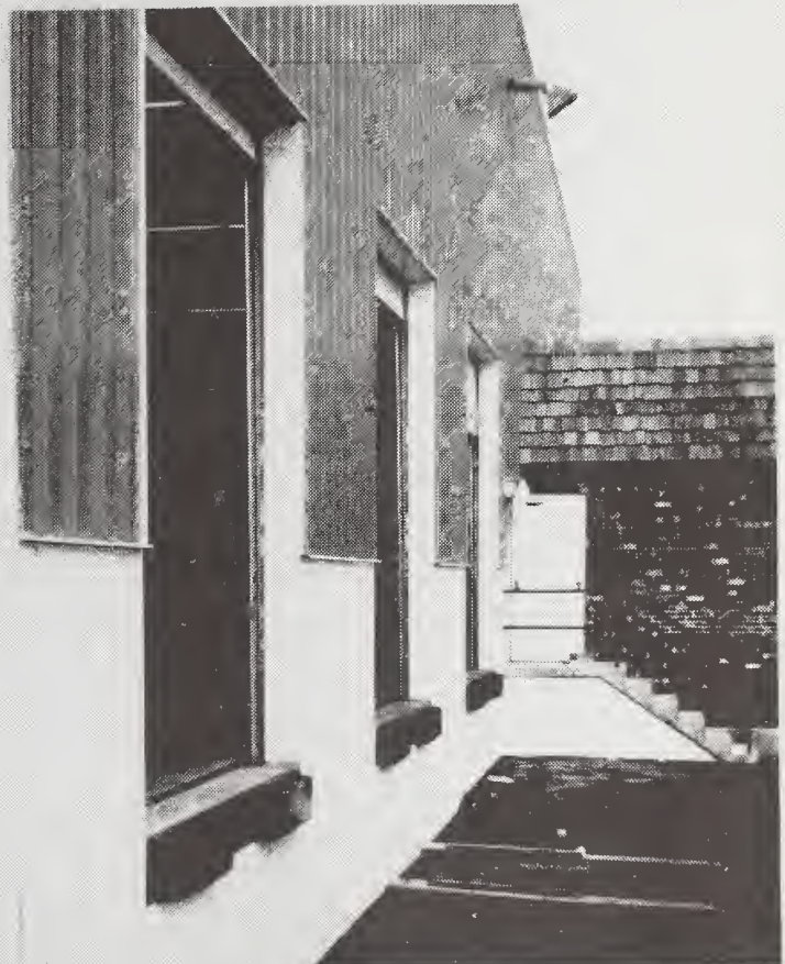
Fig. 39 - Loading dock constructed of industrial cladding and masonry. (E.2)
