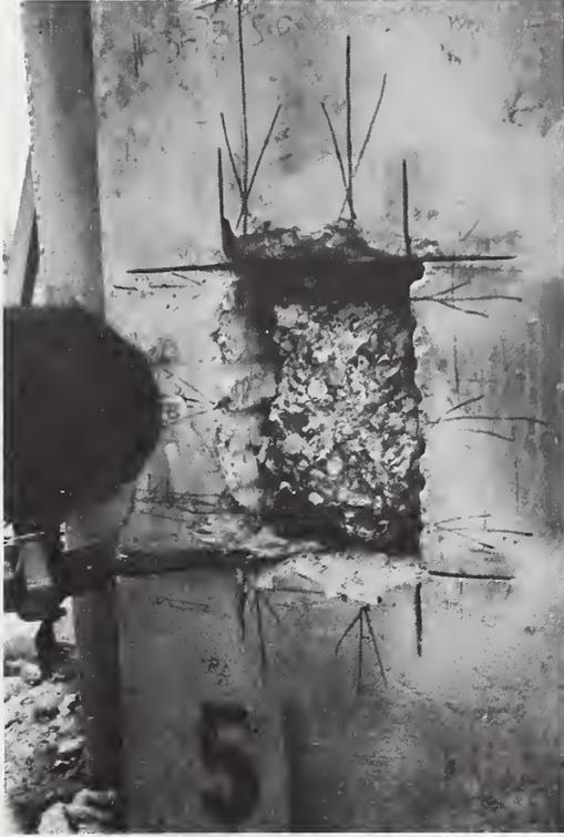
Figure 64. Chiseling Webs between Holes
