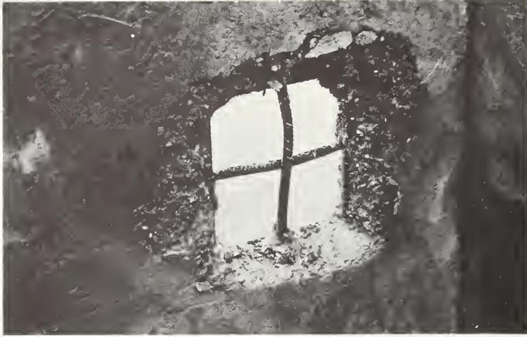
Figure 28. Interior, Slab 2, Attack A1 after Breakthrough
