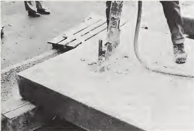
Figure 80. Stuck Jackhammer Tool Point
