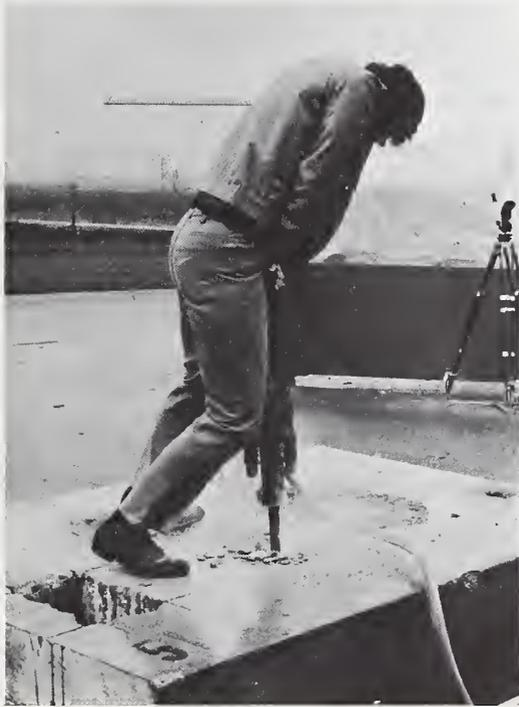
Figure 75. Pneumatic Jackhammer on Slab 5
