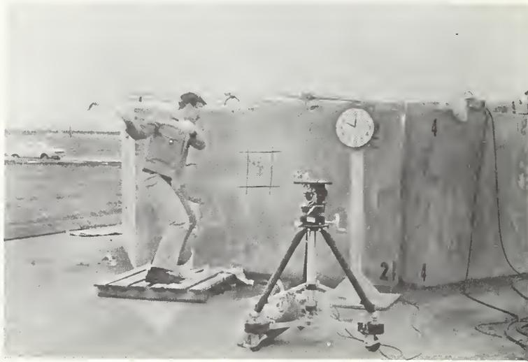
Figure 44. Hammering on Plug Left in Slab 2 by Demolition Saw
