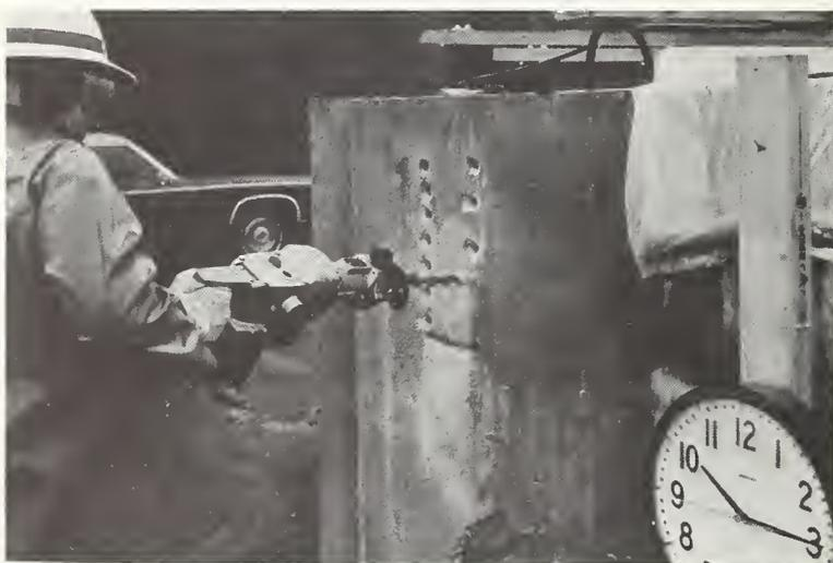
Figure 13. Drilling with Rotohammer
