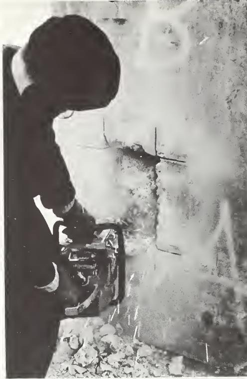
Figure 63. Sawing Reinforcing Rods
