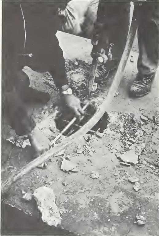
Figure 76. Opening Made by Jackhammer
