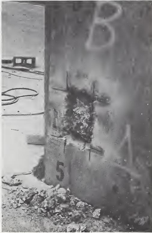
Figure 62. Material Chiseled Out of Plug
