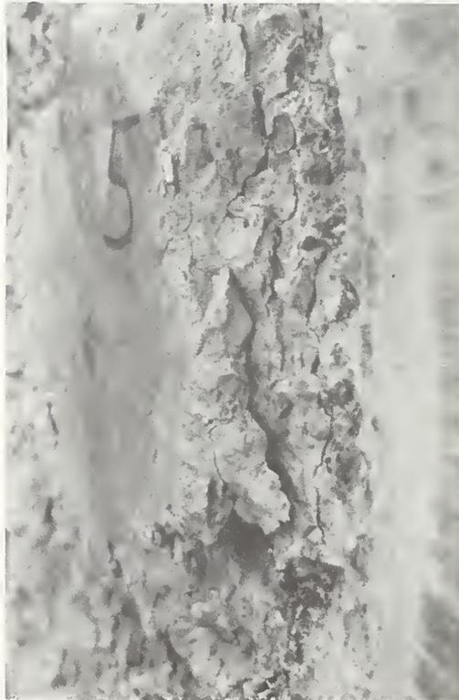
Figure 68. Close-up of Exterior Spalling
