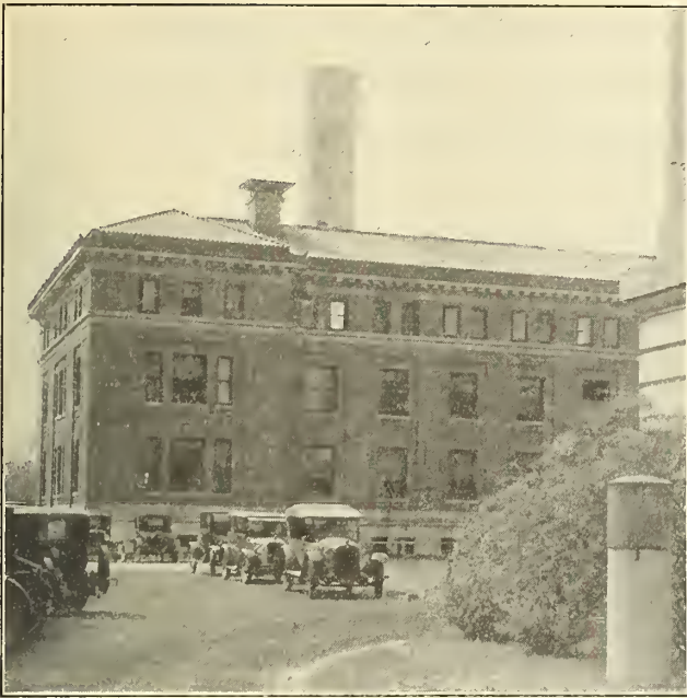
Experimental stack, 10 feet in diameter, 30 feet high, erected for measurements of wind pressure in natural winds
