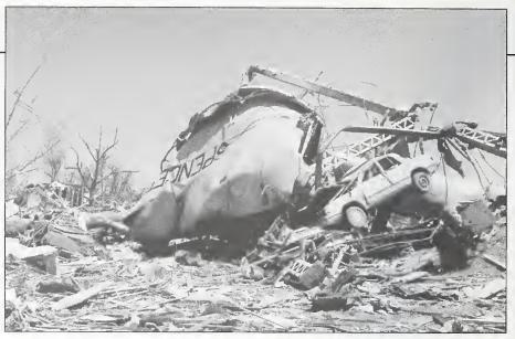
Collapsed steel water tower in Spencer, South Dakota due to the May 30, 1998 Spencer tornado.
