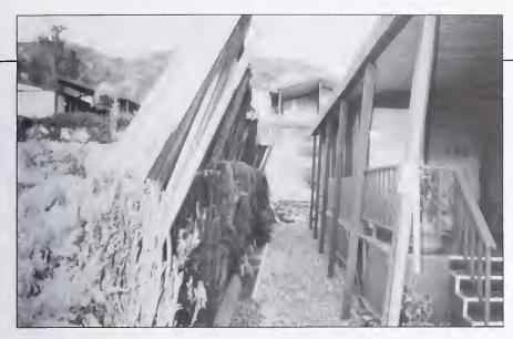
A collapsed carport shields a house from the adjacent structure that burned down completely.
