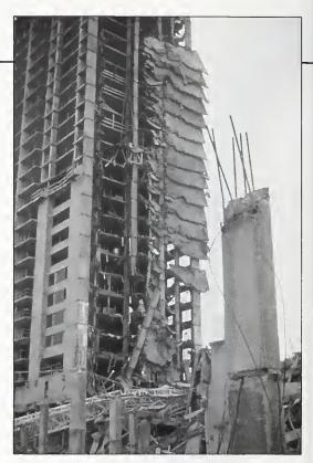
The progressive collapse of this apartment building under construction was triggered by the failure of an upper story floor as a result of premature removal of formwork.
