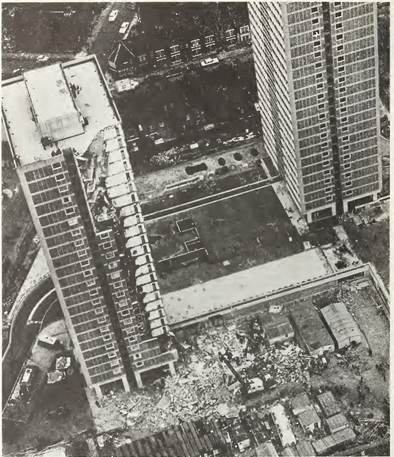
FIGURE 1. Ronan Point Apartment Building after the collapse , with a second identical building in the background. (Courtesy of London Express News and Feature Services).
