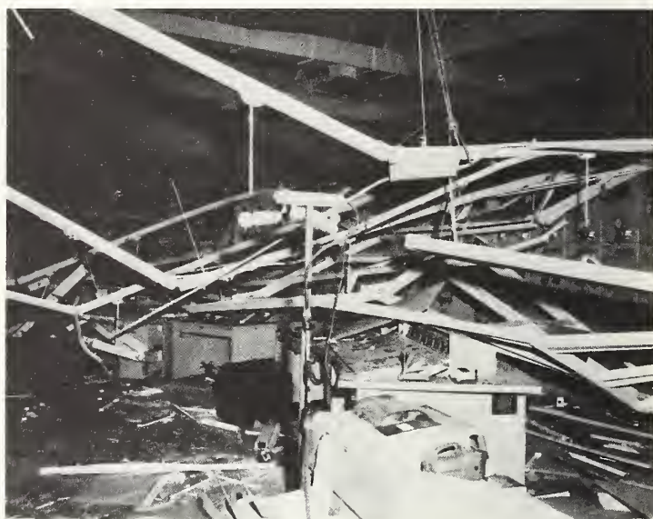
FIGURE 10. THIS SUSPENDED CEILING, LOCATED IN THE CONTROL ROOM OF A LARGE ELECTRICAL POWER FACILITY, COLLAPSED DURING THE EARTHQUAKE, INJURING ONE MAN. WHILE LITTLE DAMAGE TO CONTROL CONSOLES AND EQUIPMENT WAS REPORTED, THE FALLEN CEILING HINDERED EMERGENCY OPERATIONS.
