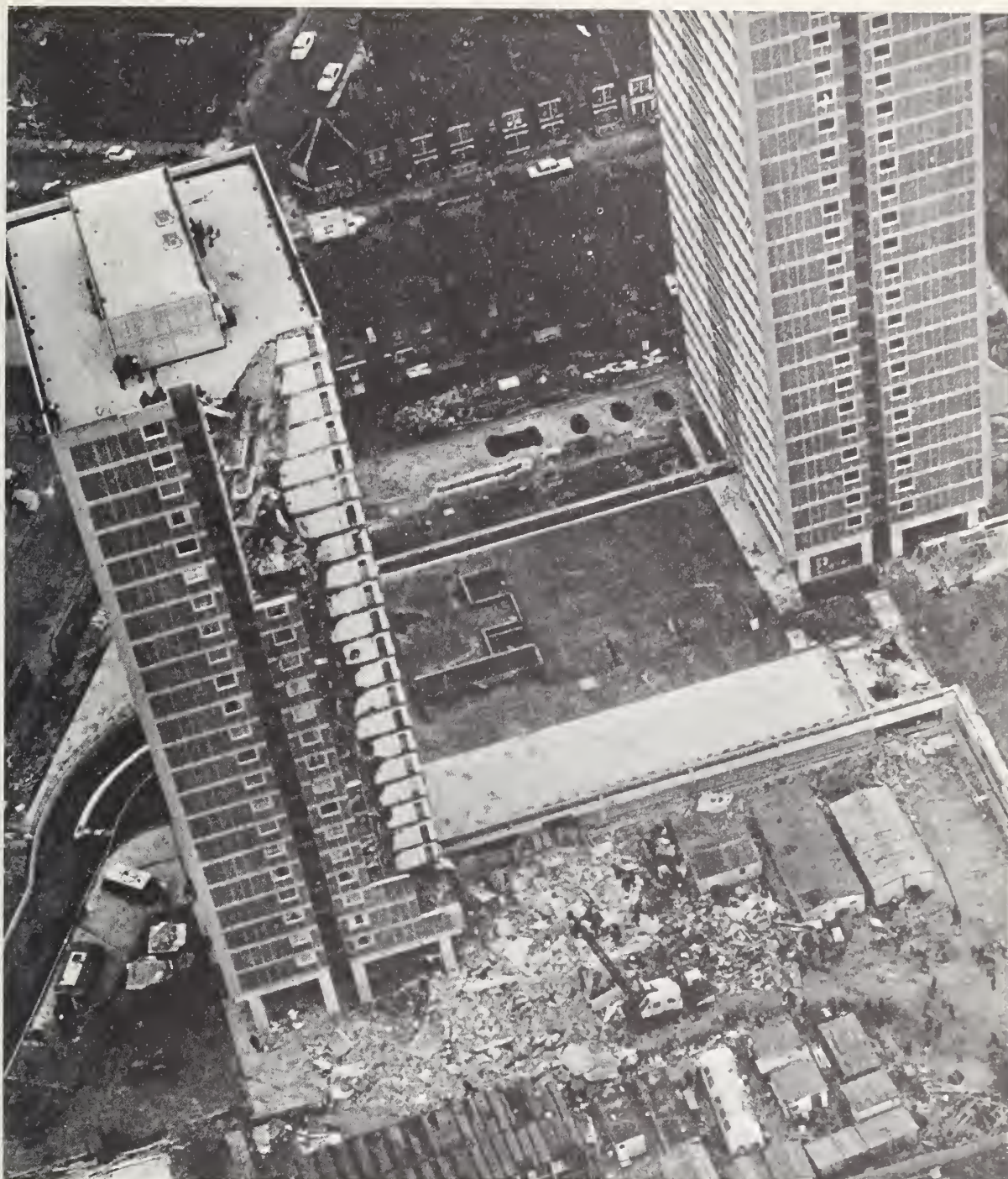
Figure 2 Ronan Point apartment building after the collapse, with a second identical building in the background. Reproduced from [1].
