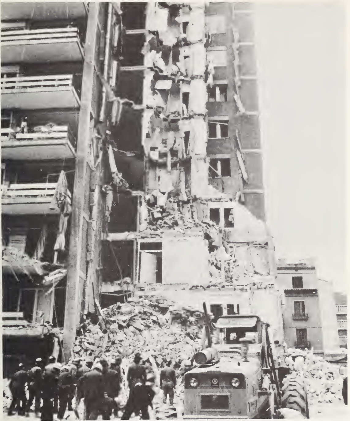
Figure 8 Apartment building at Calle Santa Amelia, Barcelona, Spain following a progressive collapse on March 6, 1972.
