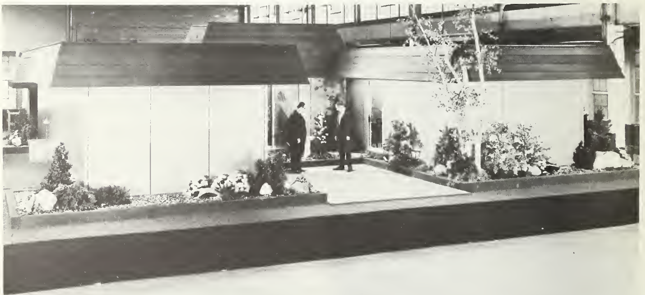
FIGURE 3. Single family house constructed with steel-faced sandwich panels.
