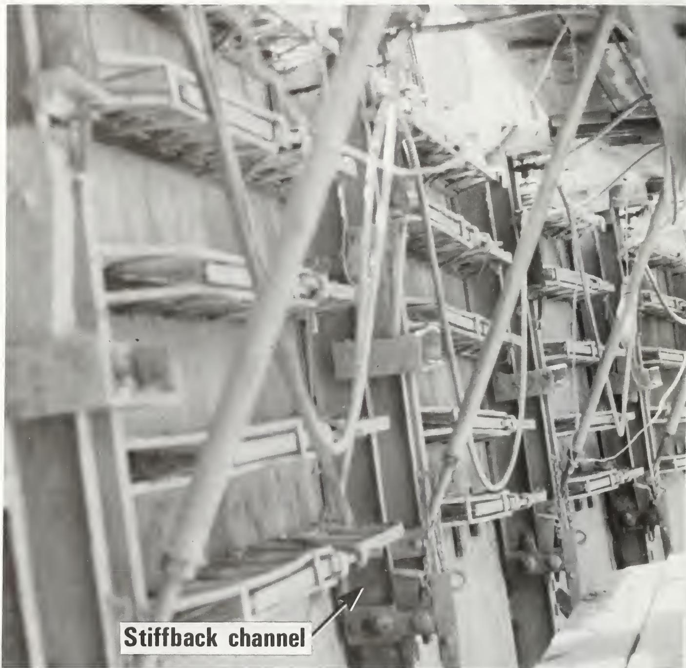
Figure 2.10 Formwork support system
