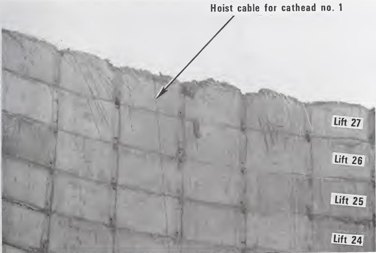
Figure 3.2 Top of Lift 27 Showing Jagged Edge
