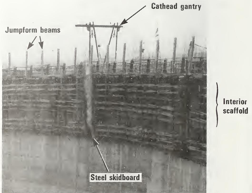
Figure 2.4 Interior View of a Tower Under Construction
