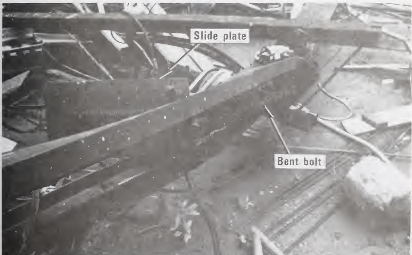
Figure 3.14 Displaced Slide Plate of Cathead Gantry No. 6
