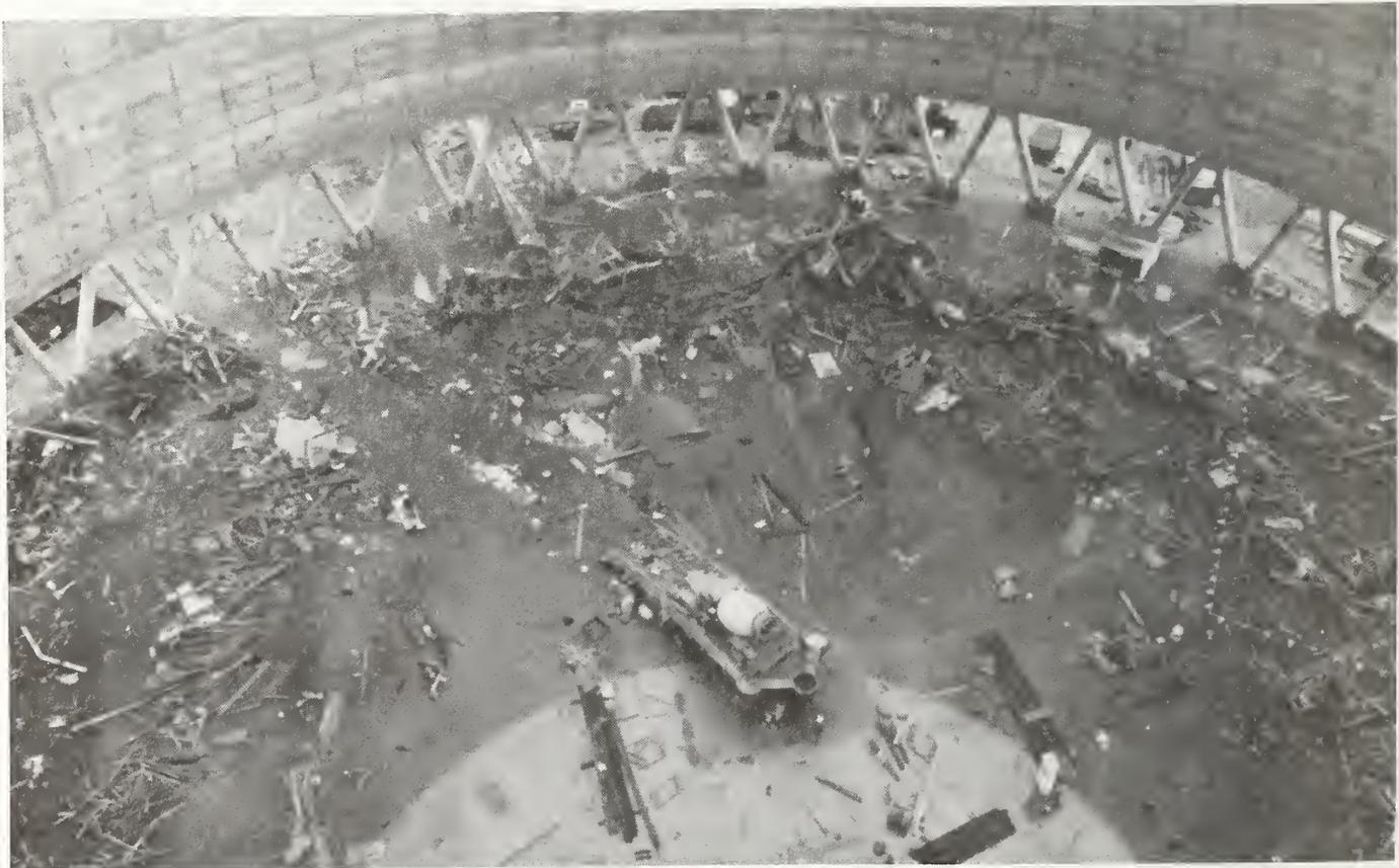
Figure 3.4 Distribution of Debris Around the Base of the Tower
