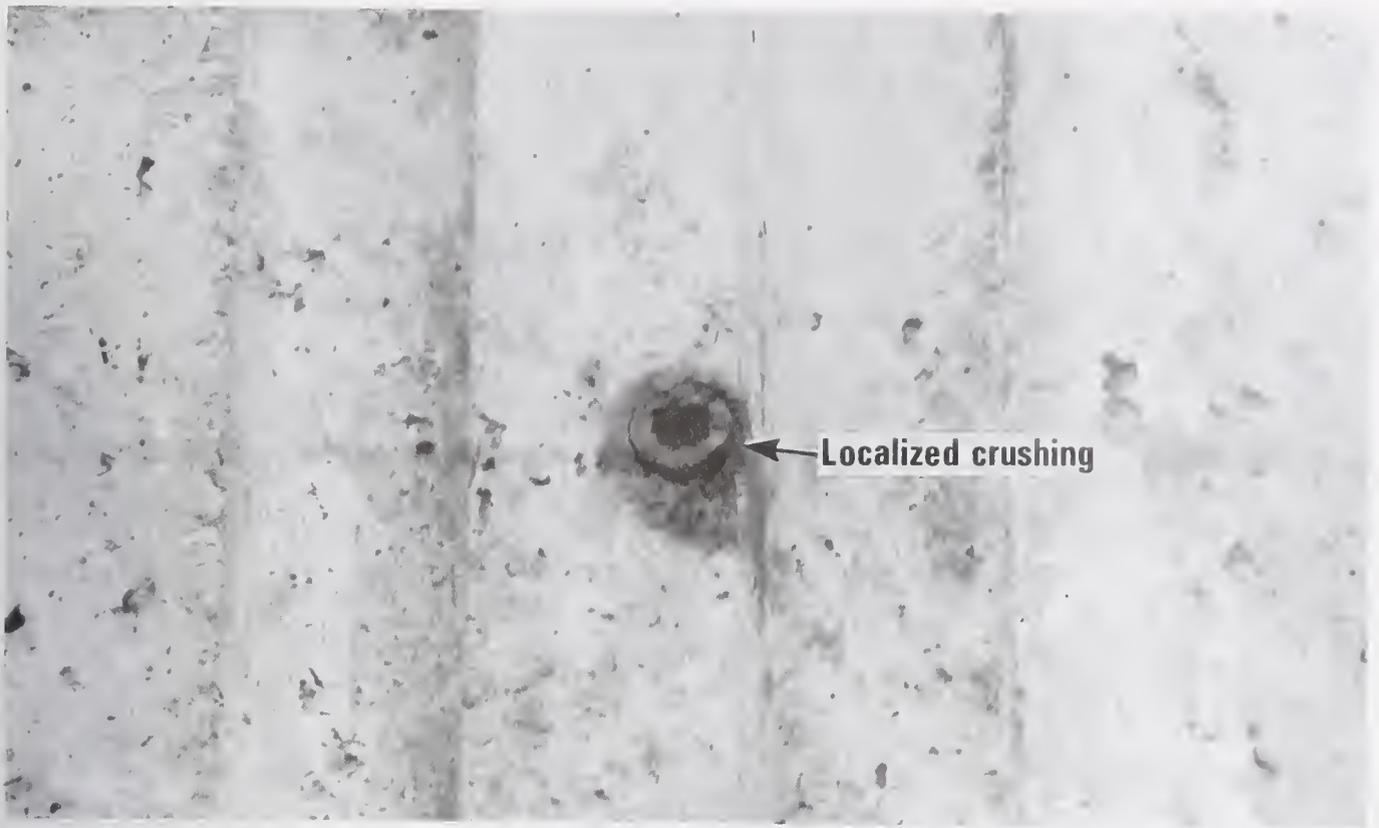
Figure 3.9 A Close-up View of the Bottom Bolt in Lift 27 Which Supported a Cathead Gantry
