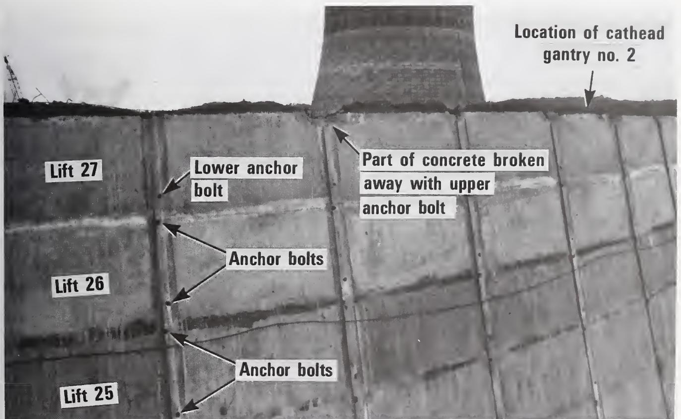
Figure 3.6 Exterior View of Top Portion of the Shell Between Cathead Gantry No. 1 and No. 2
