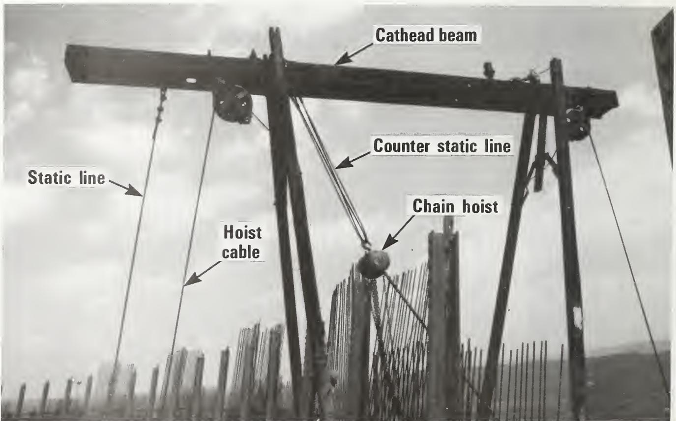
Figure 3.12 An Overall View of Cathead Gantry
