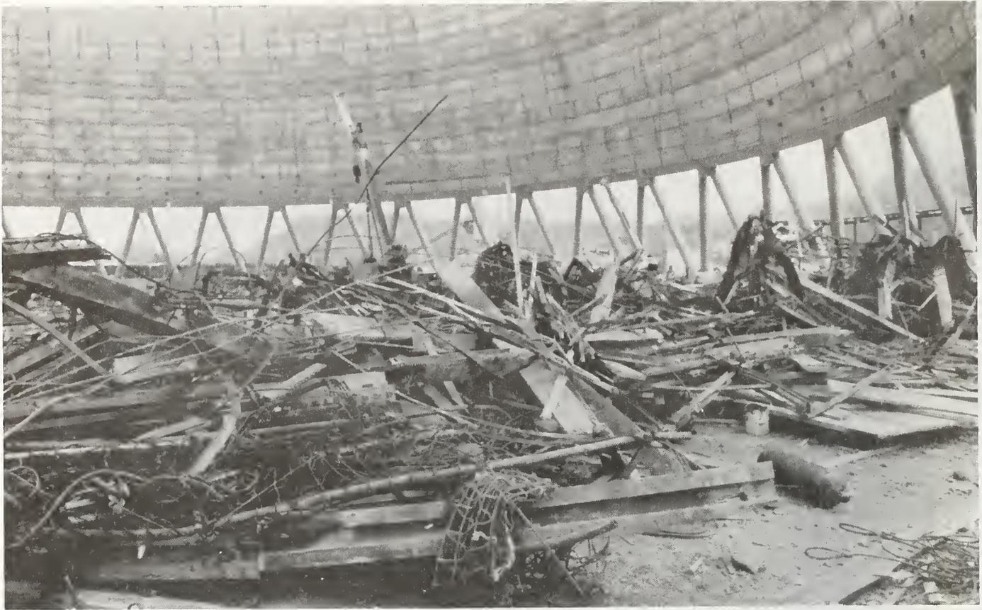
Figure 3.3 Debris Piled up Inside the Tower
