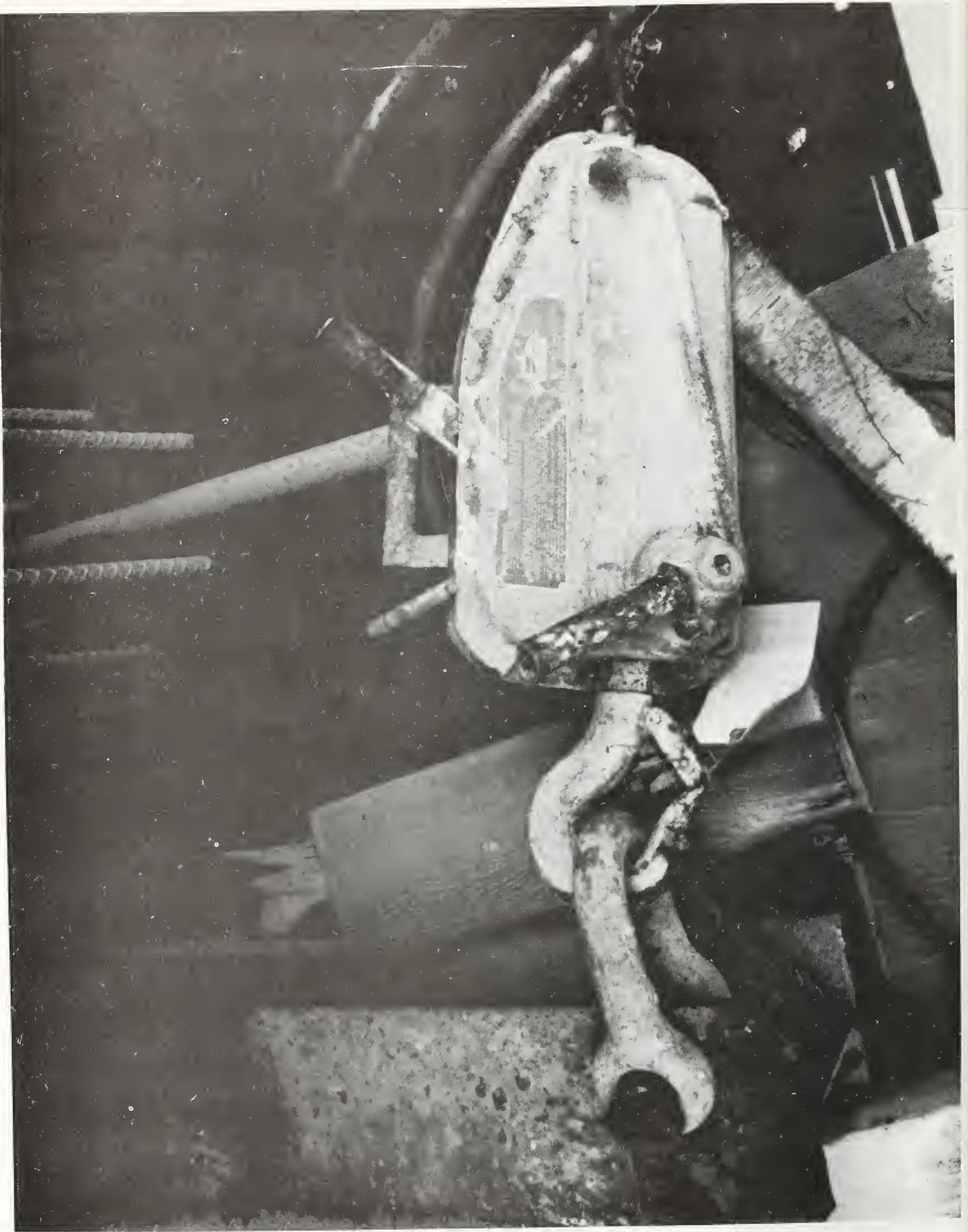
Figure 4.15 Anchorage of static line to ground through grip-hoist
