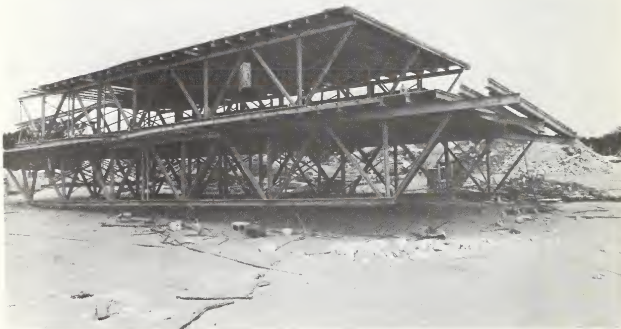
Figure 2.8 Flying forms from the two north bays recovered after the collapse
