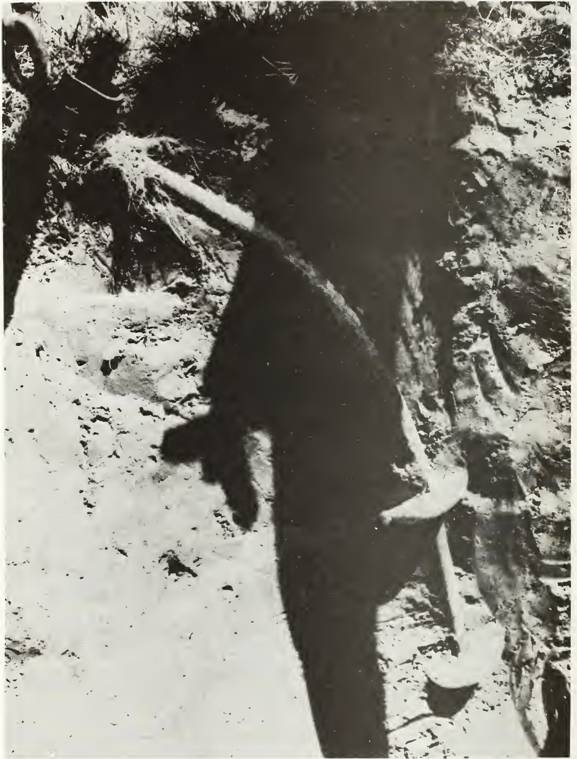
Figure 4.7 Anchor deformation in inclined test on vertically installed 4-in double helix anchor
