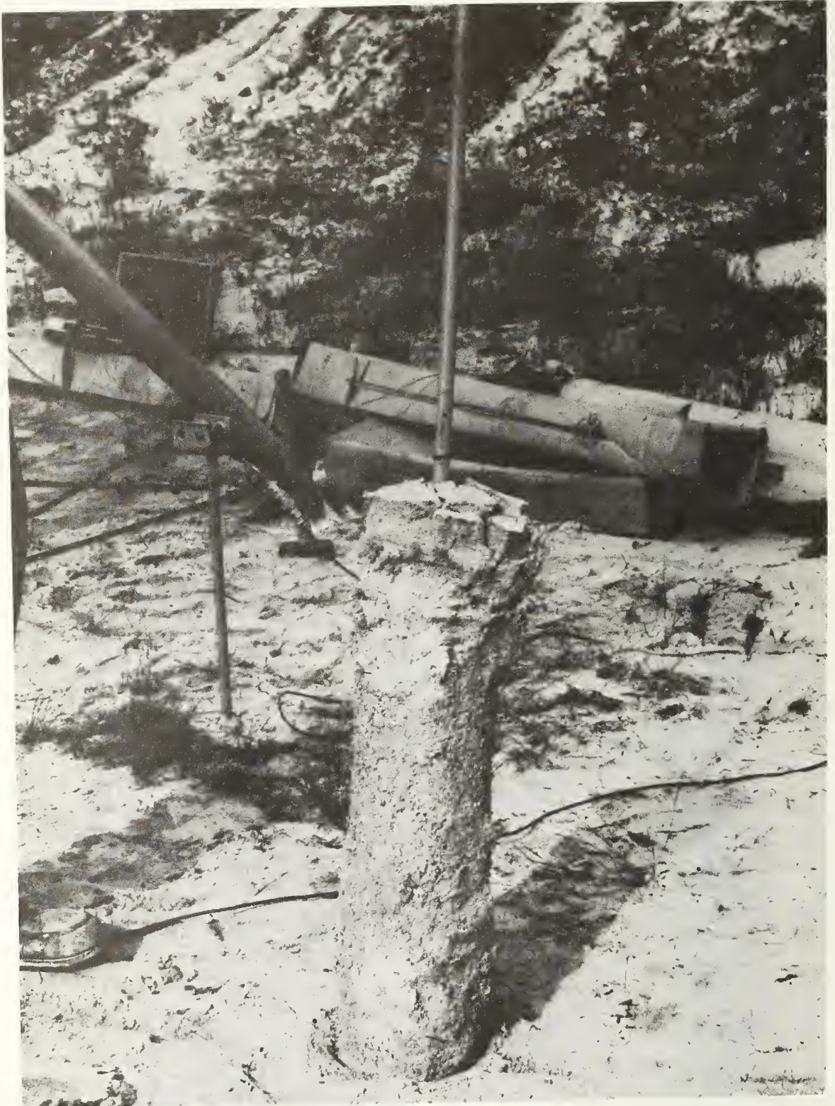
Figure 4.24 3 ft deep 6-in single helix anchor after pullout on the sandy site
