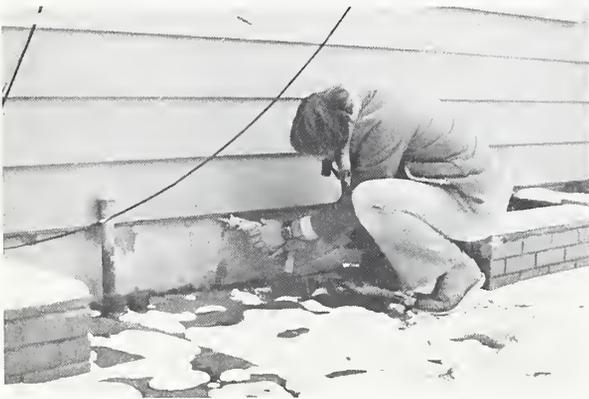
FIGURE 3. Caulking compound being applied to foundation sill.
