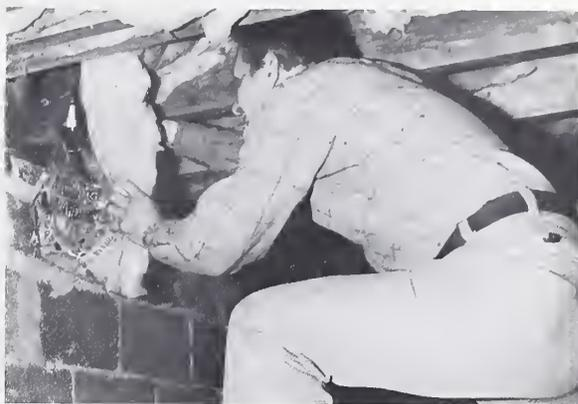
FIGURE A-7. Glass-fiber batts being installed under the floor in the crawl space.
