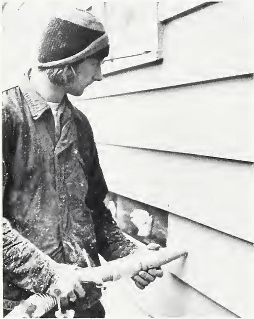
FIGURE A-3. Cellulosic fiber being blown into the walls of the test house.
