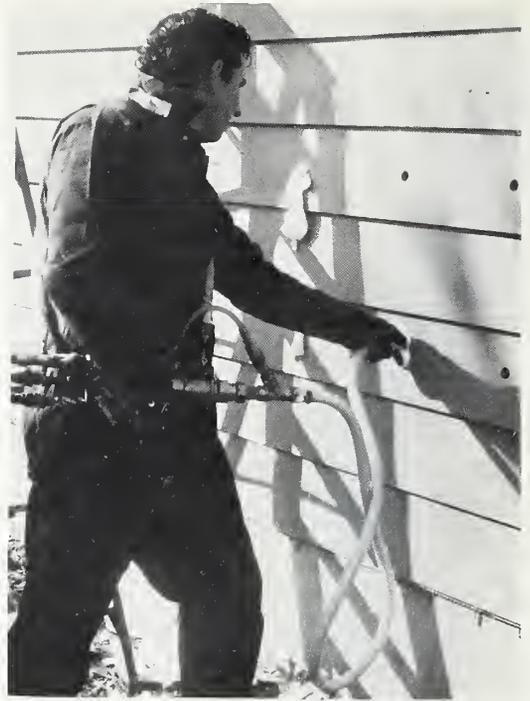
FIGURE A-5. Urea-formaldehyde foam being blown into a wall section.
