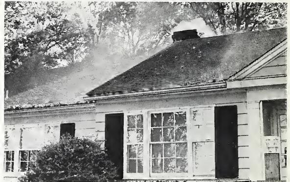
FIGURE C-4. Major air leakage path through the chimney.
