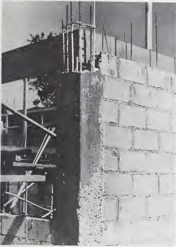
FIGURE 21 CONCRETE COLUMNS WITH CONCRETE MASONRY INFILL WALLS BEING CONSTRUCTED FOR SINGLE FAMILY DWELLING OCCUPANCY IN CENTRAL LUZON, THE PHILIPPINES.
