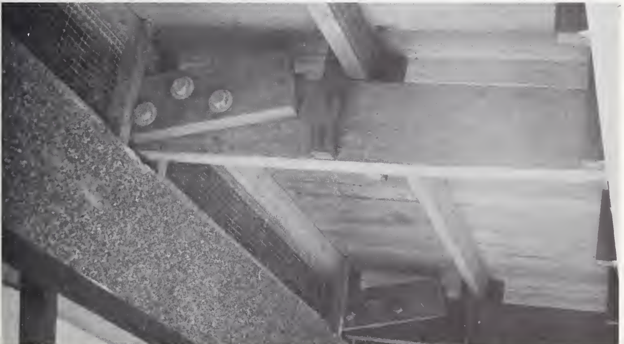
FIGURE 48 CEILING JOIST BOLTED TO RAFTERS RESISTS OUTWARD THRUST OF RAFTER; WOOD CLEATS TIE PURLINS TO RAFTERS.
