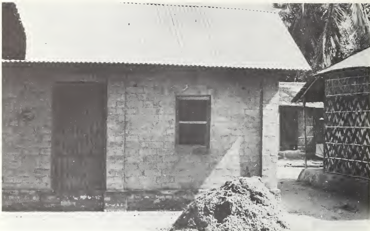
FIGURE 27 CARE SPONSORED HOUSING PROJECT NEAR DACCA, BANGALADESH SHOWING CINVA-RAM WALL CONSTRUCTION WITH CORRUGATED METAL ROOFING.
