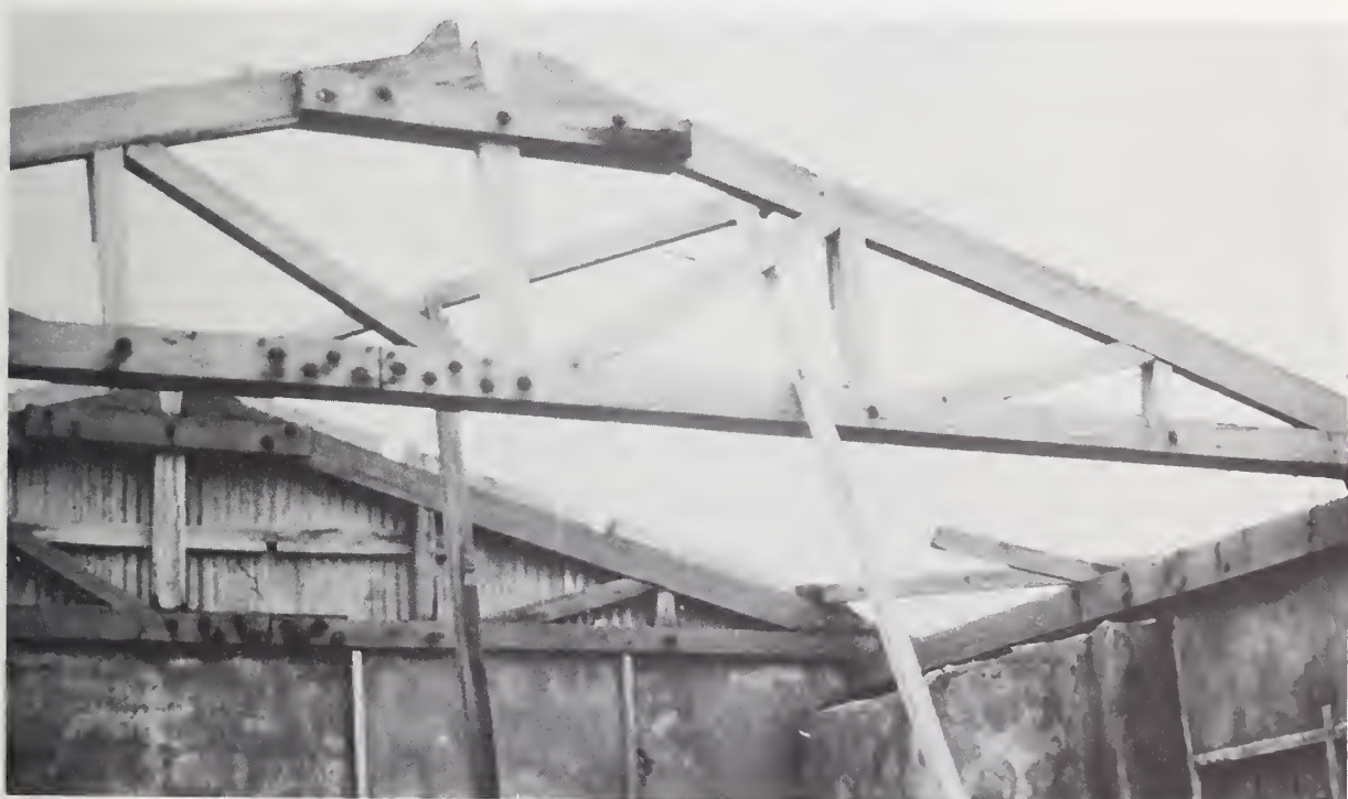
FIGURE 52 STAINING FROM CORROSION OF BOLTS AND NAILS.
