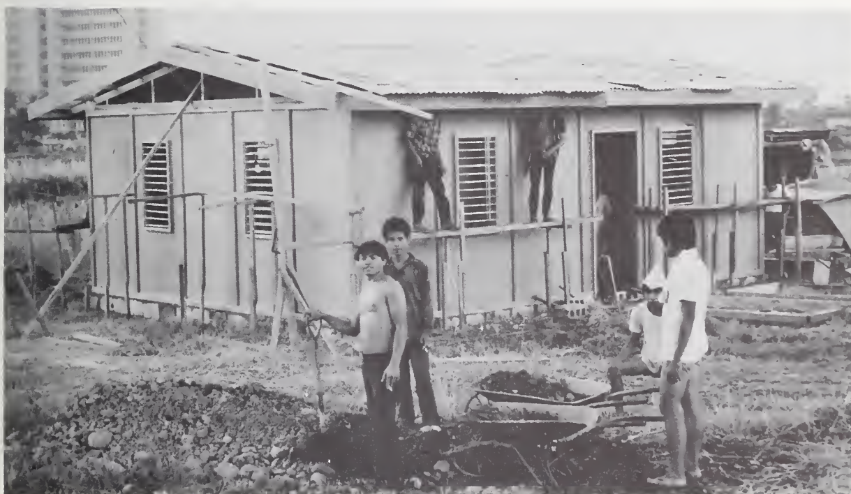
FIGURE 40 WOOD-FRAME WALL AND ROOF.
