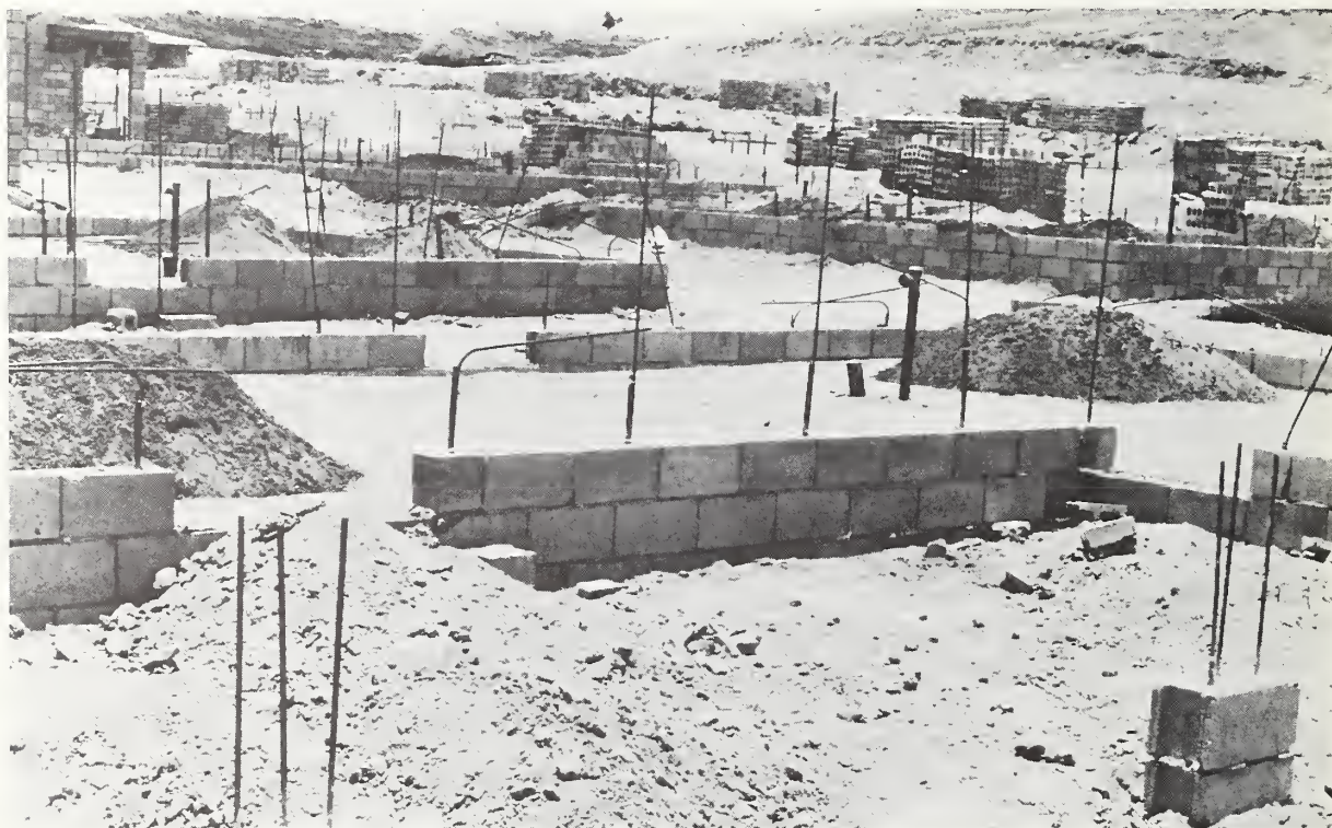
FIGURE 24 REINFORCED CONCRETE MASONRY WALLS UNDER CONSTRUCTION FOR HOUSING IN CENTRAL LUZON, THE PHILIPPINES.
