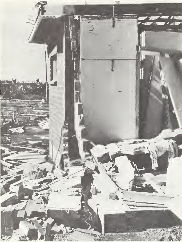
FIGURE 16 BUILDING IN DARWIN, AUSTRALIA SHOWING PARTIAL COLLAPSE OF ROOF AND MASONRY INFILL WALLS CAUSED BY THE DECEMBER 1974 CYCLONE.
