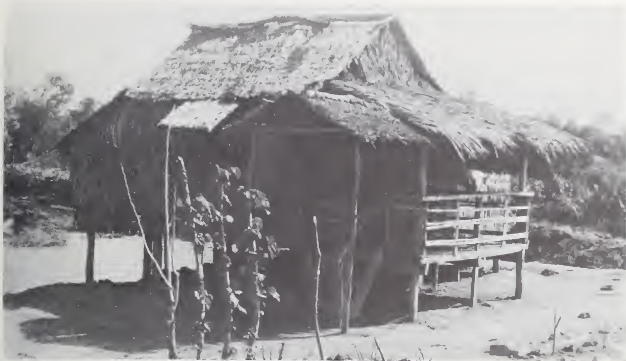
FIGURE 39 POLE-TYPE CONSTRUCTION.
