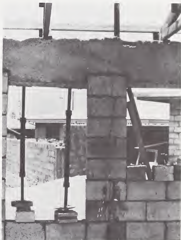
FIGURE 26 SINGLE FAMILY HOUSING UNDER CONSTRUCTION IN CENTRAL LUZON, THE PHILIPPINES, SHOWING CONCRETE BOND BEAM DETAIL OVER OPENINGS.
