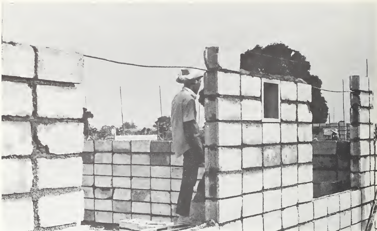
FIGURE 19 STACKED BOND CONCRETE MASONRY WALL CONSTRUCTION FOR SINGLE FAMILY OCCUPANCY IN CENTRAL LUZON, THE PHILIPPINES.
