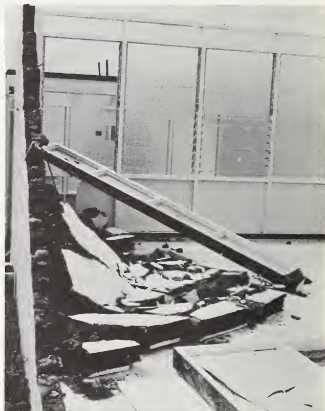
FIGURE 12 SINGLE FAMILY HOUSE SHOWING COLLAPSE OF ROOF AND EXTERIOR WALL DURING THE PHILLIPINES TYPHOON IN NOVEMBER 1970.
