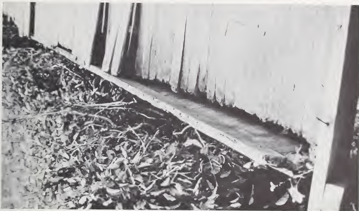
FIGURE 51 JOINT FAILURE DUE TO DECAY IN WOOD.
