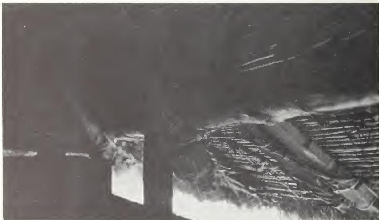
FIGURE 42 ROOF FRAMING TIED DOWN WITH STRIPS OF BAMBOO.
