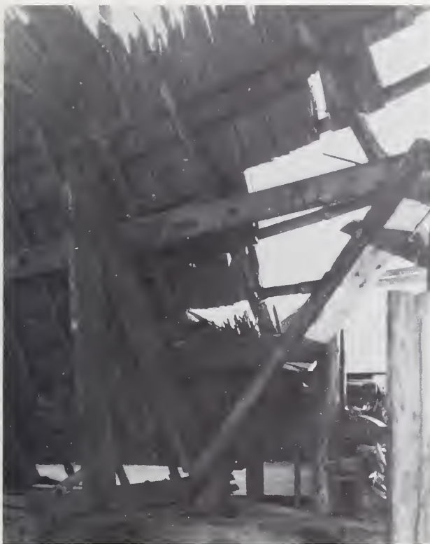
FIGURE 43 THATCH ROOF WITH THATCH PARTIALLY BLOWN OFF.
