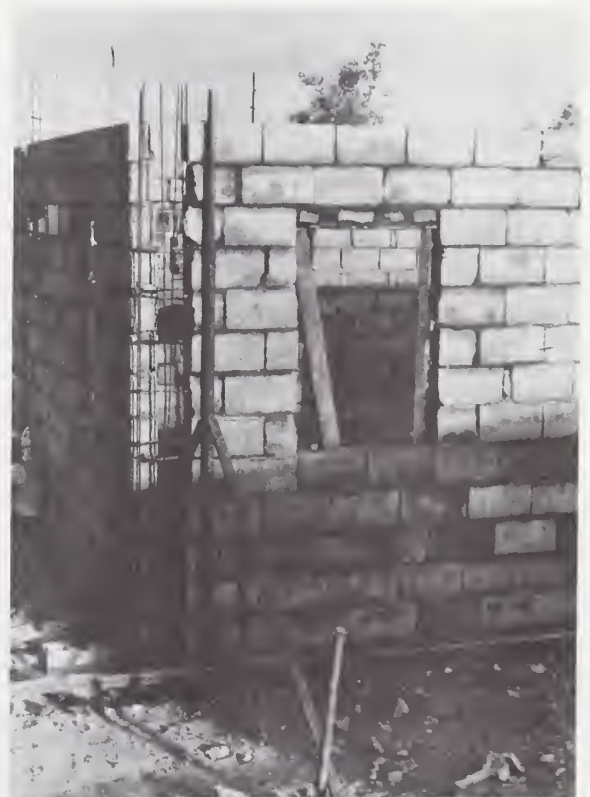
FIGURE 22 CONSTRUCTION OF SINGLE FAMILY HOUSING UNIT IN CENTRAL LUZON THE PHILIPPINES, SHOWING CONCRETE MASONRY FILLER WALLS AND REINFORCEMENT OF CORNER COLUMN.
