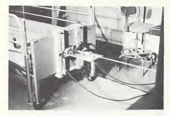
FIGURE 2. Detail of bed, load cell, and connections.
