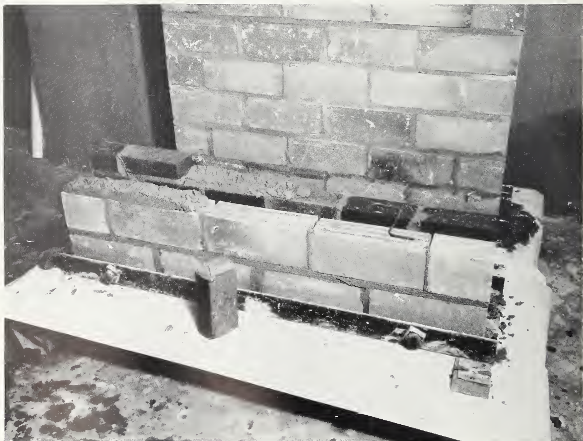
FIGURE 12.—Brick-faced cavity wall, workmanship M.
