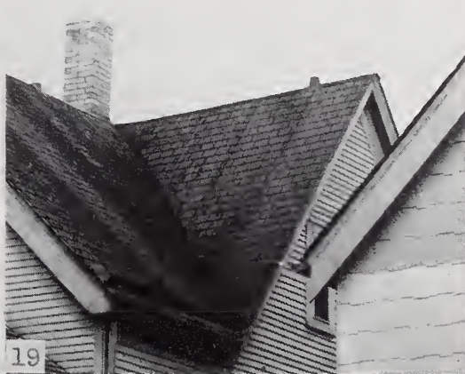
FIGURES 14 to 19.— Mineral-surfaced, asphalt-prepared roll roofings.
