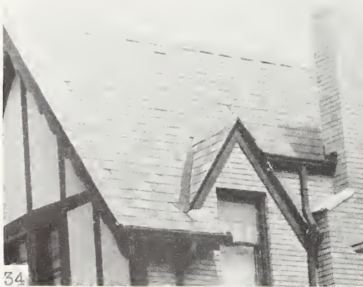
FIGURES 32 to 37.—Cement-asbestos shingles and slate.
