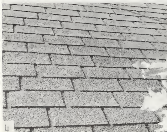
FIGURES 2 to 7.— Asphalt shingles (individual shingles applied by the American method).
