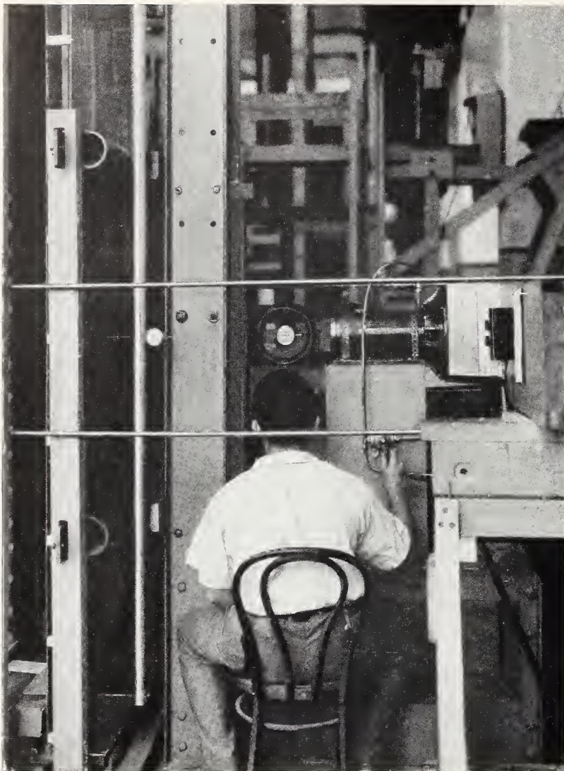
FIGURE 10.—Wall specimen CQ-T5 under transverse load.
