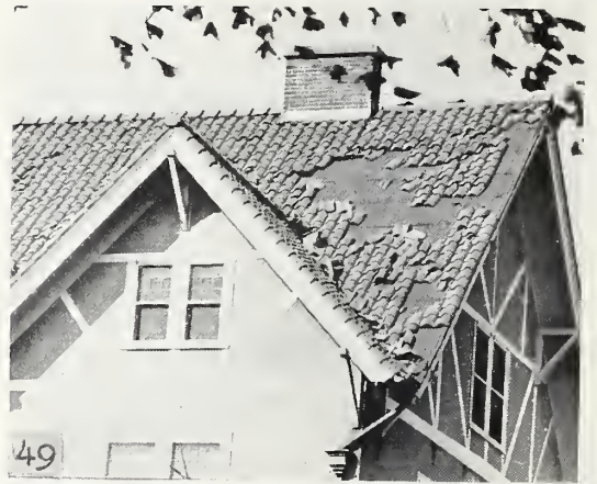
FIGURES 44 to 49.—Hurricane damage to roofs.
