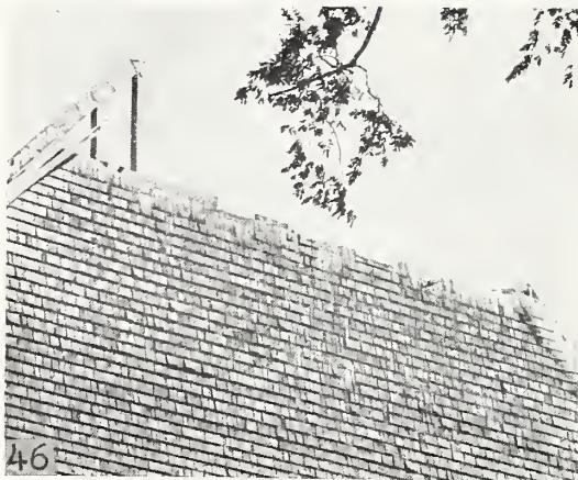
FIGURES 44 to 49.—Hurricane damage to roofs.
