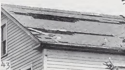
FIGURES 38 to 43.— Metal roofs, flashings, and hurricane damage to asphalt shingles.
