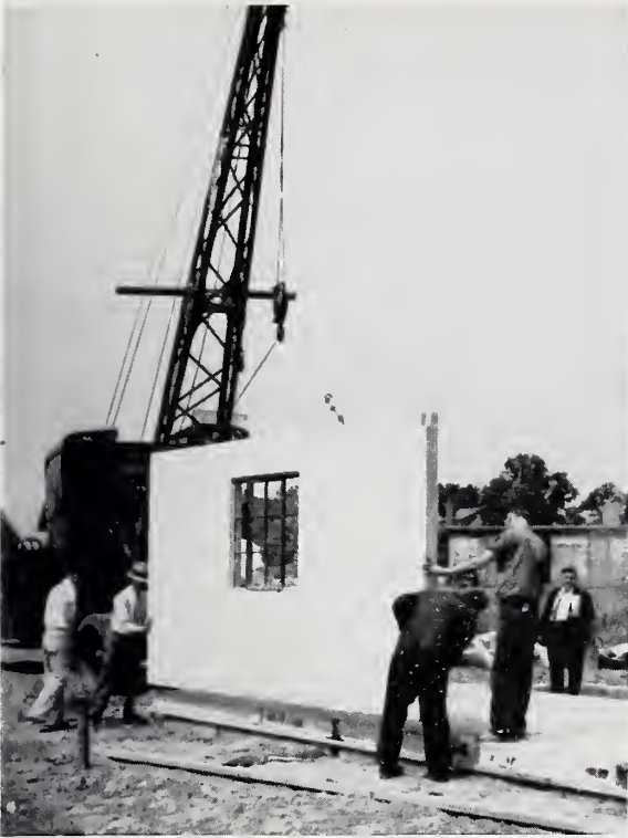
FIGURE 20.—Erecting "Twachtman" wall panel by means of a crane truck.
