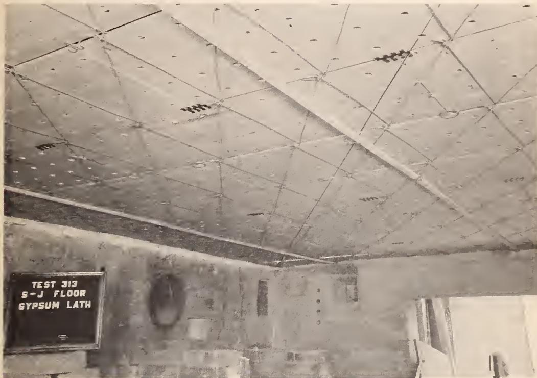
FIGURE 4. *Lathed ceiling with diagonal wire reinforcing.*
