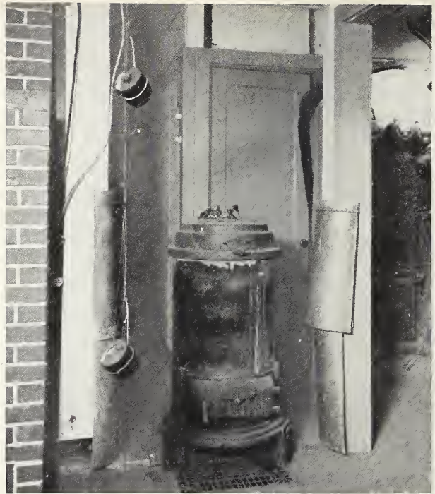
FIGURE 16. Heater A in position 4 over floor grill used in conjunction with underfloor plenum.
