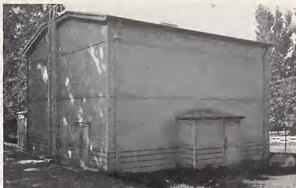
FIGURE 4. Insulated enclosure for the Test Bungalow.
