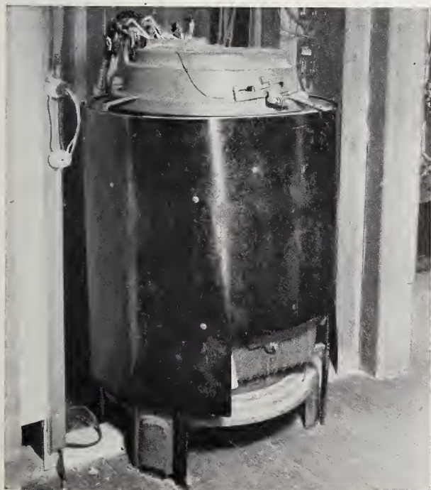
FIGURE 9. Heater A with jacket 4 in position 4 in temporary opening in partition wall.
