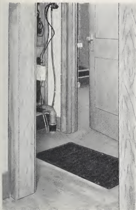
FIGURE 7.—Single gas-burning floor furnace, gravity type, shown from above the floor.
