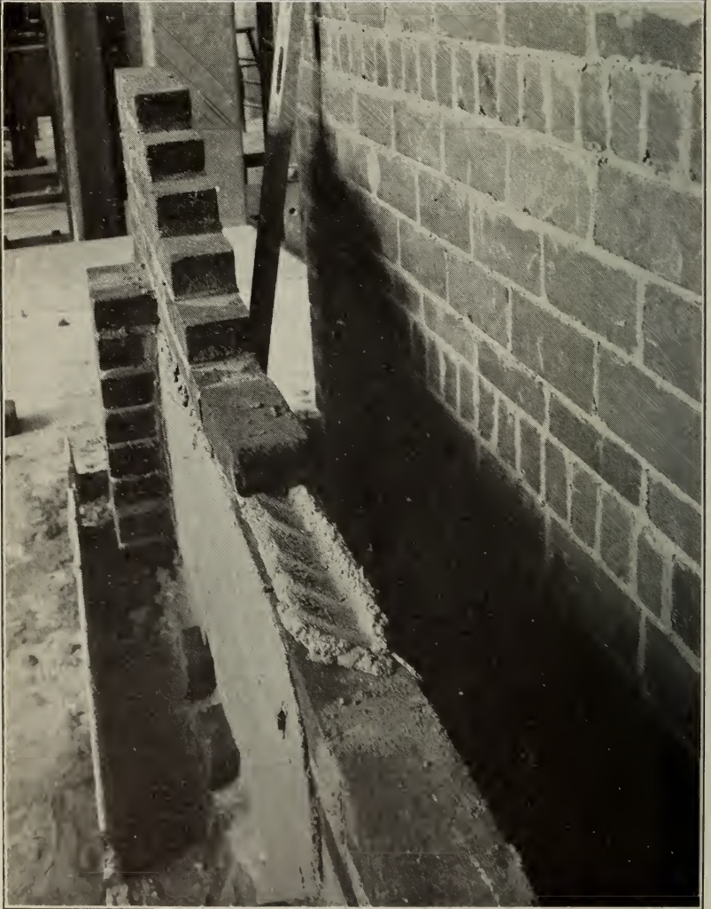
FIGURE 7.—View showing furrowed horizontal joints
