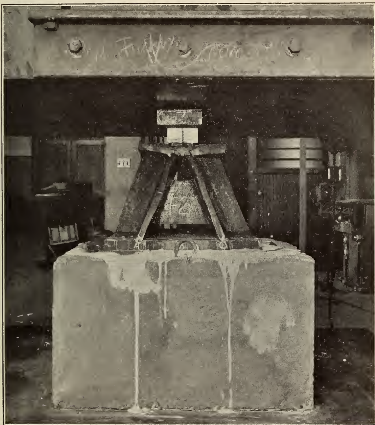
FIGURE 5.—Pedestal F_2 in the 10,000,000-pound capacity testing machine after test
