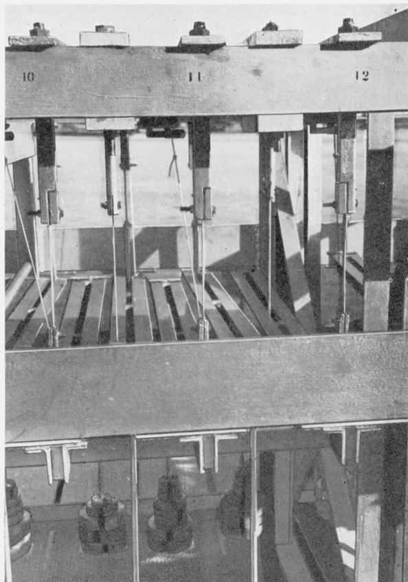
FIGURE 3.—Stressed and unstressed specimens in marine-atmosphere stress-corrosion rack.
