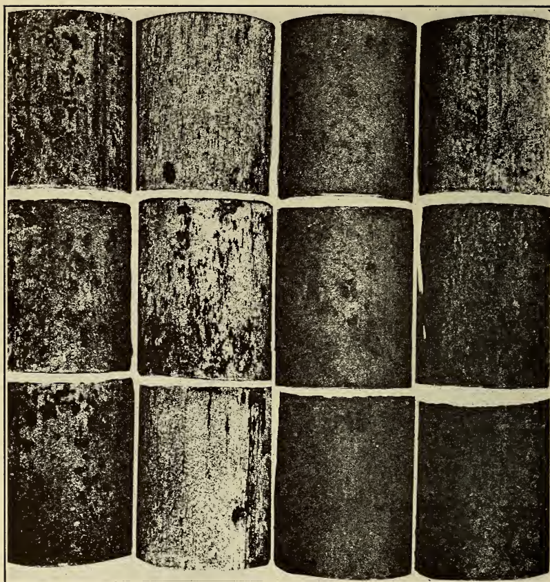
FIGURE 13.— Appearance of the outer surface of wrought-iron pipe after corrosion
