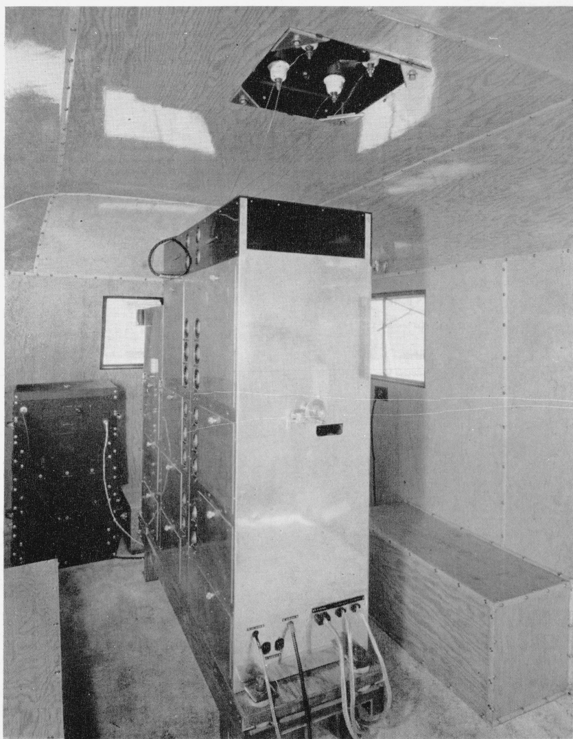
FIGURE 10.—Interior of trailer, showing transmitter as installed for both transportation and operation.
