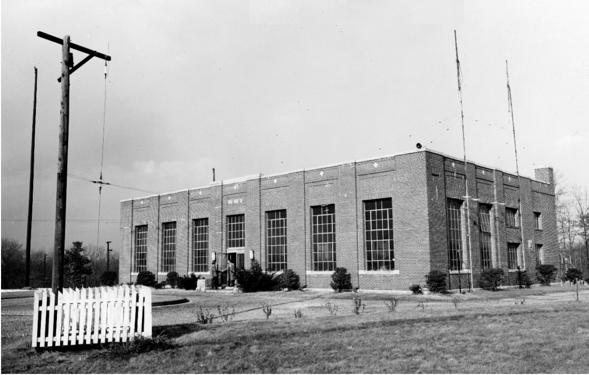
Fig. 13. WWV building, with dipole antenna on the left.
