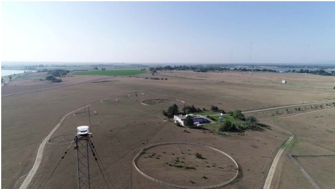
Fig. 26. Aerial view of the WWV site with the 2.5 MHz antenna in the foreground.
