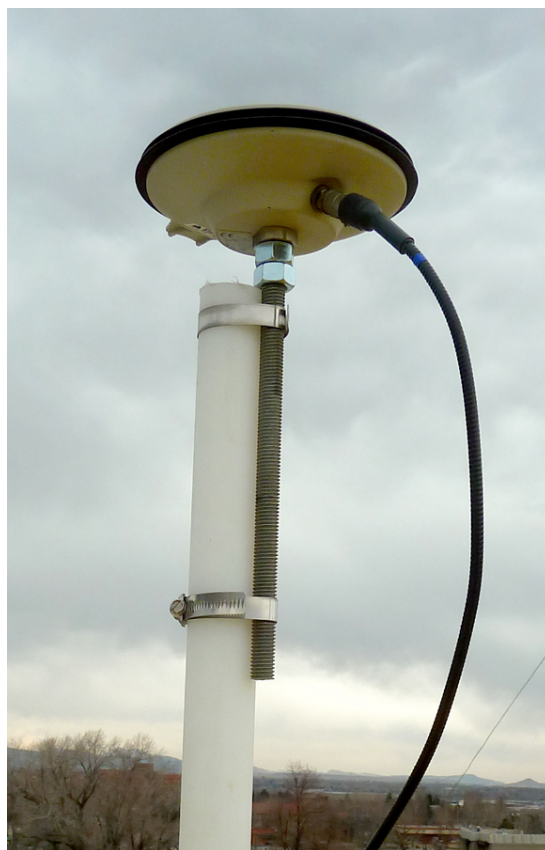
Fig. 3. GPS antenna mounted on rooftop location.
