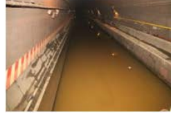
Source: MTA. (November 2, 2012) Water in Cranberry Tube on AC Line.
