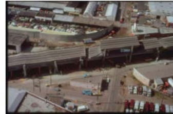
Source: NOAA/NGDC, E.V. Leyendecker, USGS, Collapse of Freeway in 1989 Loma Prieta, CA Earthquake
