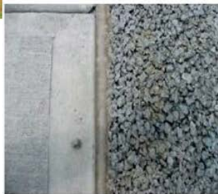
Figures 23: Pilot - Porous Concrete Sidewalk at DEP's Paerdegat Basin CSO Detention Facility
