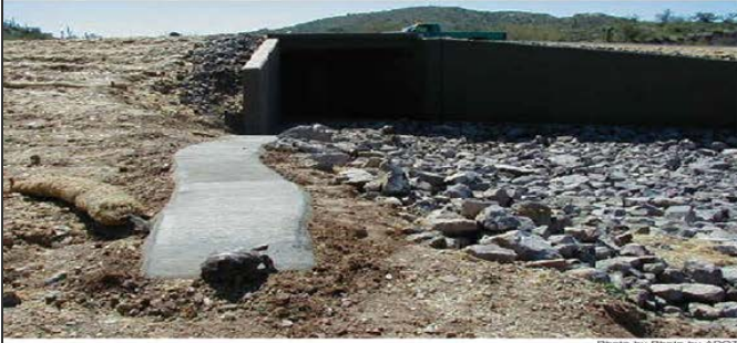
Photo by Photo by ADOT In Arizona, baby tortoises no longer fall into riprap in front of culverts, thanks to ramps
