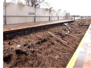
Source: MTA. Debris from Jamaica Bay fills Tracks Inside Broad Channel A Station on November 1, 2012.
