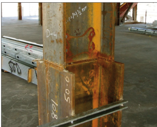
Figure 7-3. Steel special moment frame complete joint penetration groove weld column splice.
