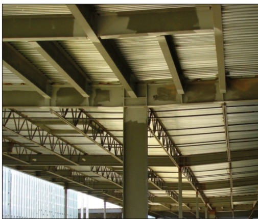
Figure 5-2. Stability bracing using transverse framing.
