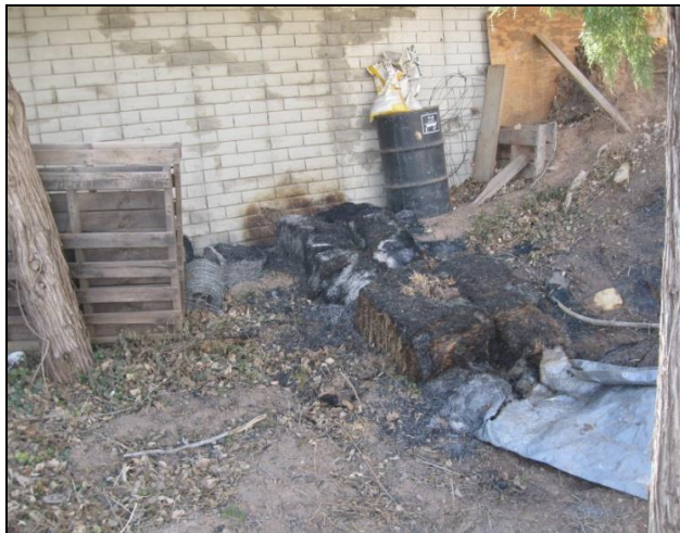
Figure 33 Burned hay bales leading from destroyed secondary structure to primary structure causing scorching on the brick siding. Categorization of defensive actions is unknown, NIST photo.
