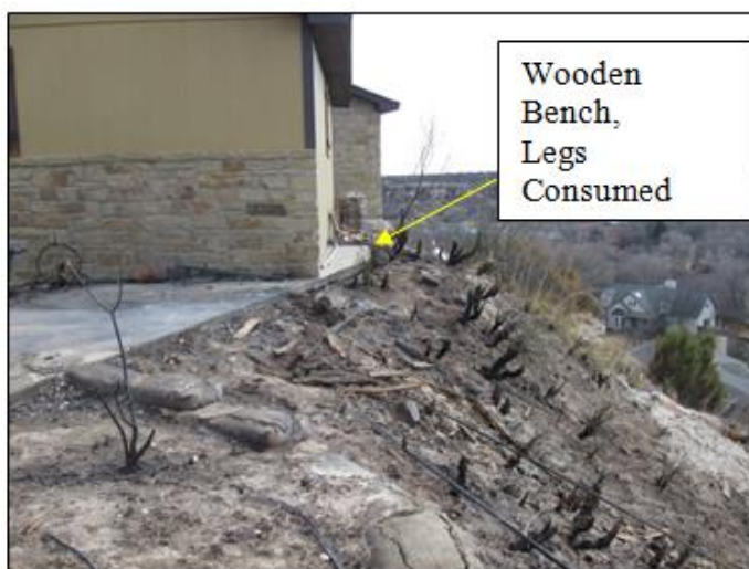
Figure 56 Damaged wooden bench and burned and unburned vegetation on west side of 100 Camino Alto, NIST photo.
