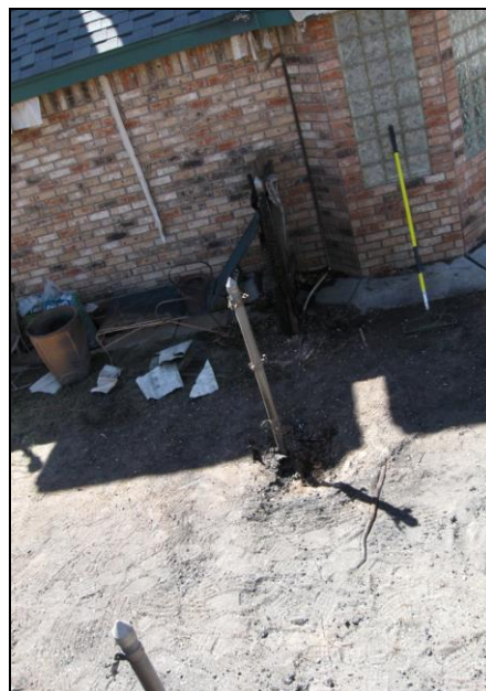
Figure 57 Partially destroyed wood fence, which caused scorching to brick siding and melting of vinyl soffit, NIST photo.
