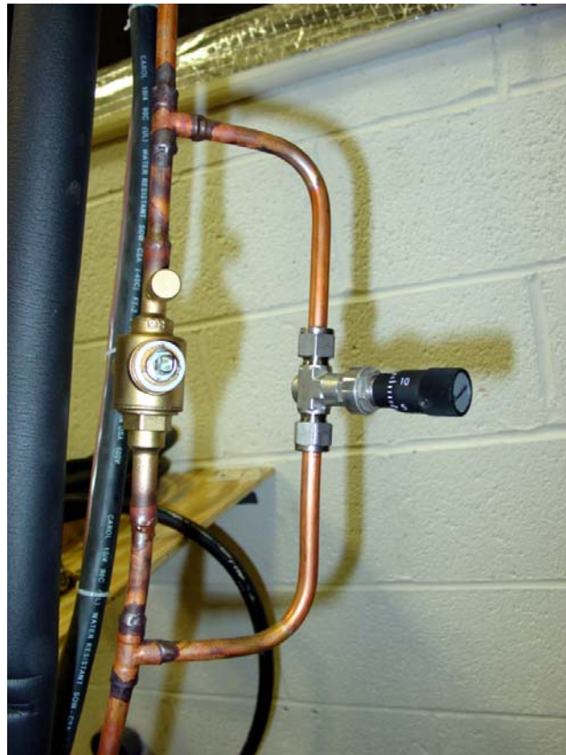
Figure 3.11. Artificial setup to implement a liquid line restriction fault using a shut-off valve and a metering valve
