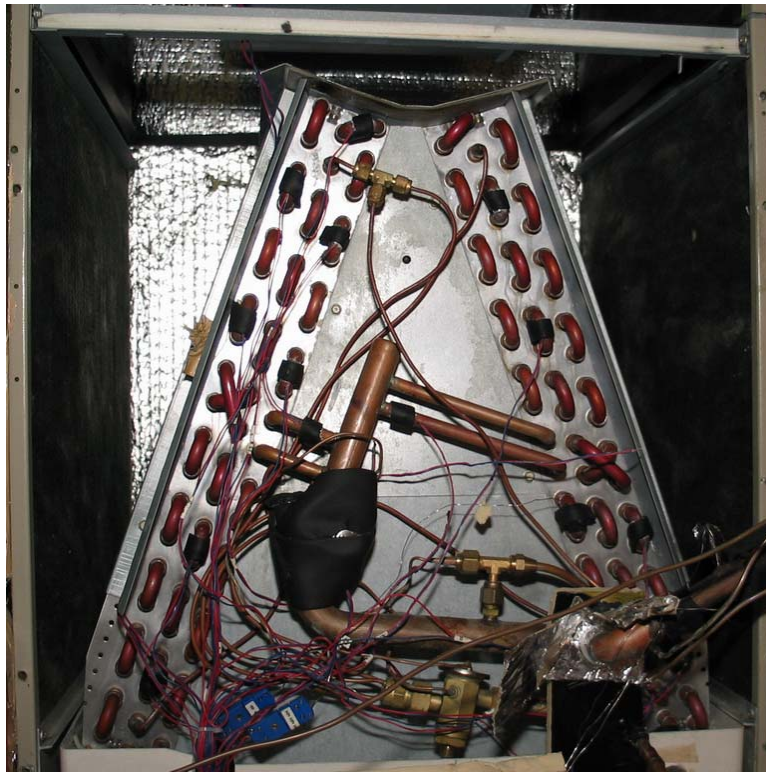
Figure 3.4. Side view of the indoor coil in an upflow configuration
