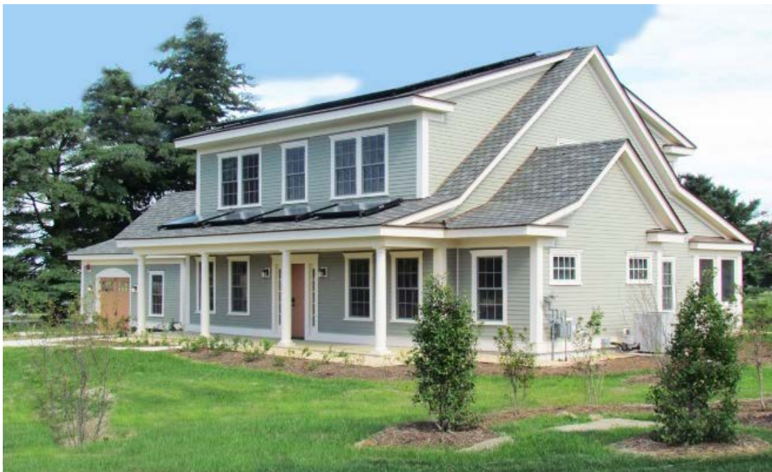
Figure 3-1 NIST Net-Zero Energy Residential Test Facility
