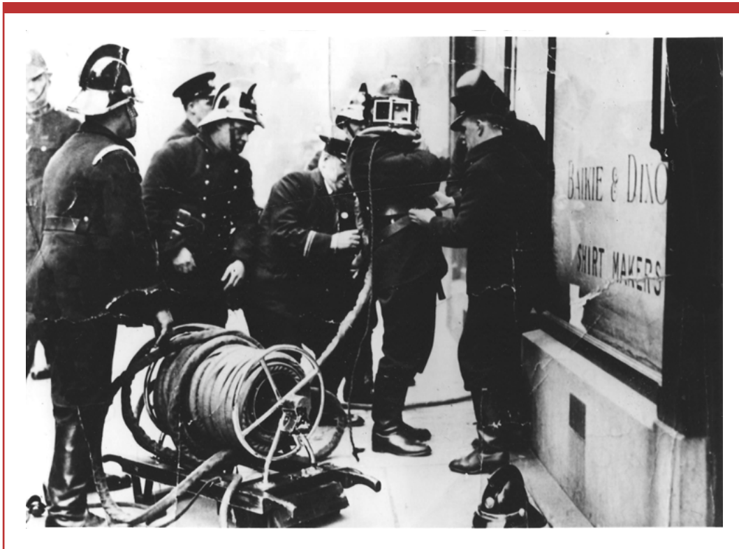
Figure 3.1 A tethered helmeted fire fighter prepares to enter a structure. (Source: Photograph from the Scottish Fire and Rescue Service Heritage Trust.)
