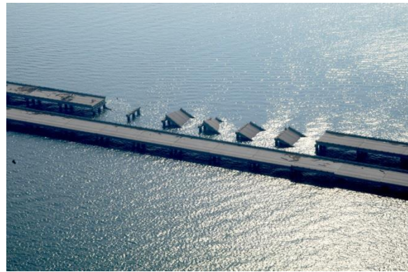
Figure 13-3: Bridge sections knocked off their supports during Hurricane Katrina due to wave action (Source: Photo by Win Henderson [FEMA 2014d])
