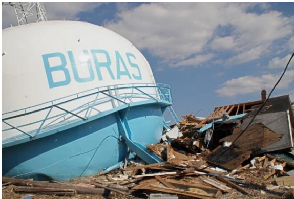
Figure 16-5: Collapsed water tank in Buras, LA near Hurricane Katrina landfall location [Source: FEMA]
