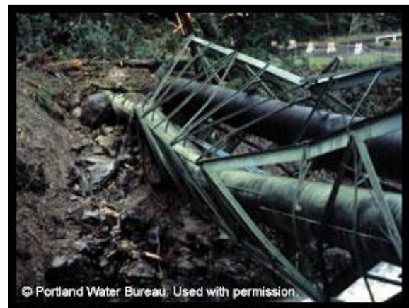
Figure 16-2: Water transmission pipeline bridge damaged by landslide
