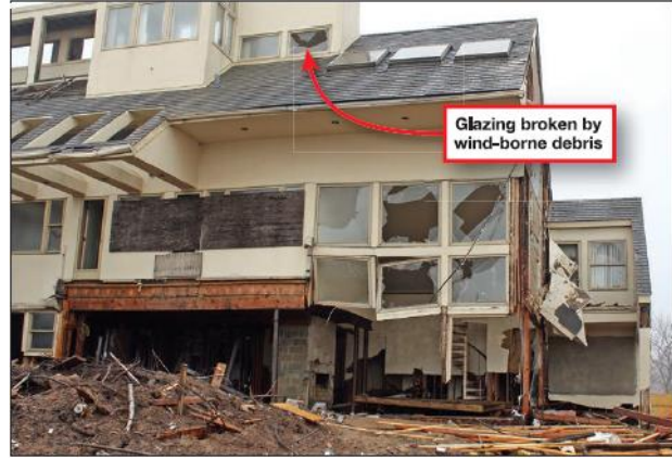
Figure 12-11: Wind and wind-borne debris resulted in considerable damage to glazing on this building. [Source: FEMA]
