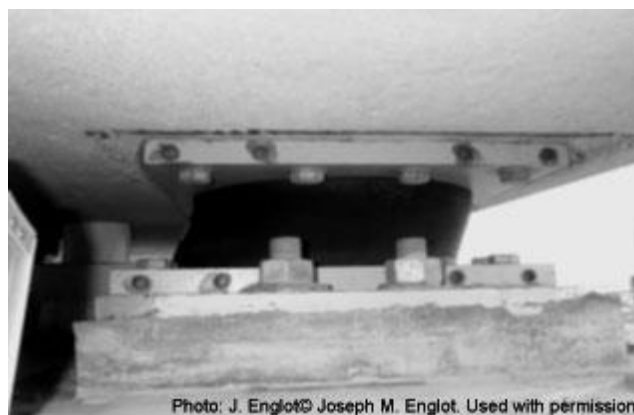
Figure 13-11: Airtrain seismic isolation bearing
