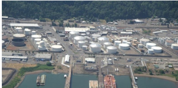
Figure 11-7: Portland, OR liquid fuel tank farm is vulnerable to failures in pipelines in Washington State. (Source: Yumei Wang [DOGAMI 2012])
