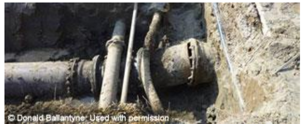
Figure 16-4: Liquefaction caused differential settlement between pile-supported structures and buried pipe during the 2011 Tohoku Earthquake
