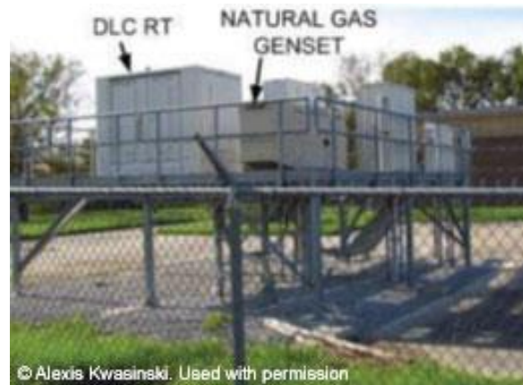
Figure 15-5: Elevated DLC RT with natural gas standby generator installed after Hurricane Katrina
