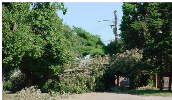
Figure 13-2: Local road blocked by fallen trees after remnants of extra-tropical storm struck Kentucky [Source: Kentucky Public Service Commission 2009]
