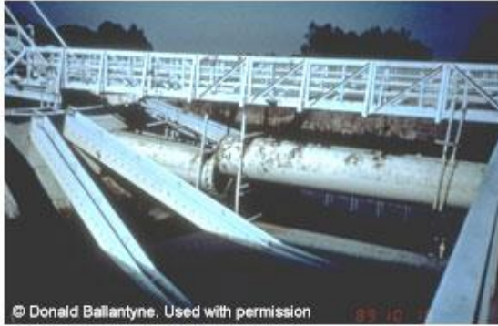
Figure 16-3: Santa Clara Valley Water District, water treatment plant clarifier launders damaged due to sloshing, 1989 Loma Prieta Earthquake
