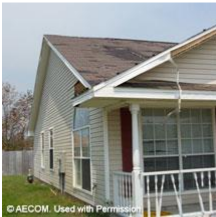
Figure 12-4: Damage to roof covering, vinyl siding and fascia as the result of wind
