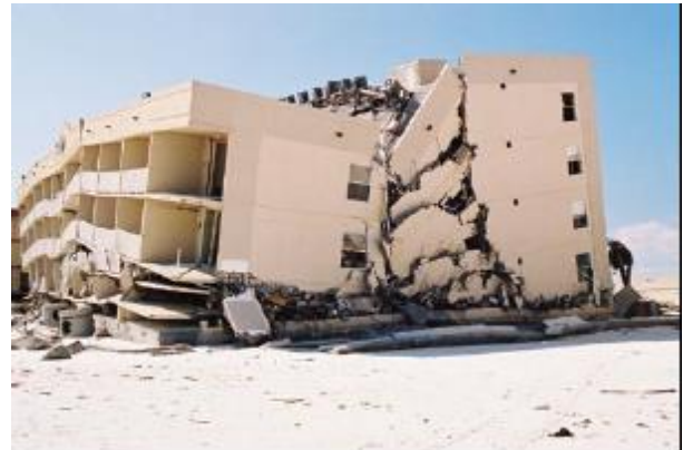
Figure 12-12: Collapse of five-story building due to undermining (from flooding) of shallow foundation [Source: FEMA]
