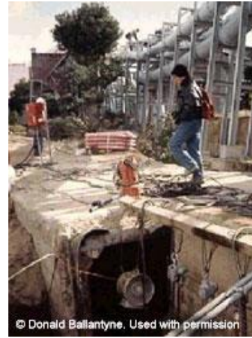
Figure 16-12: Higashinada WWTP Channel offset by liquefaction in 1995 Kobe Earthquake
