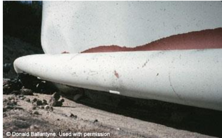
Figure 16-8: Steel tank elephant's foot buckling in 1994 Northridge Earthquake
