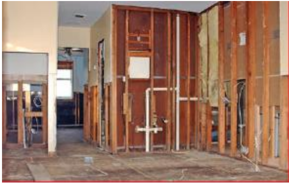
Figure 12-6: As a result of an estimated 0.9-1.2 m (3-4 ft) of flooding, interior walls had to be replaced as well as an exterior door and window [Source: FEMA]
