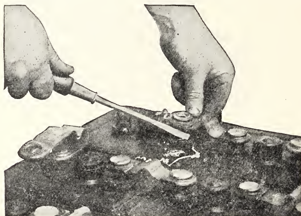
FIG. 36.— Prying off the connector after the boring-out operation shown in Fig. 35. Care must be taken in this operation not to break the cover of the jar
