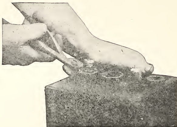
FIG. 38.— Removal of the sealing nut. The sealing nut of the post on the right has been removed and is lying beside the post. Not all makes of batteries have sealing nuts. Sealing nuts are of several different types, varying with the manufacturer
