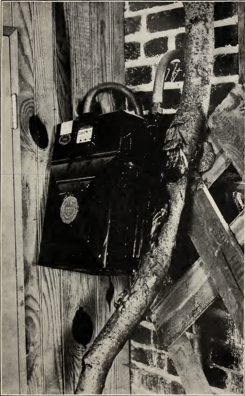
FIG. 14.—A poor gas meter installation
