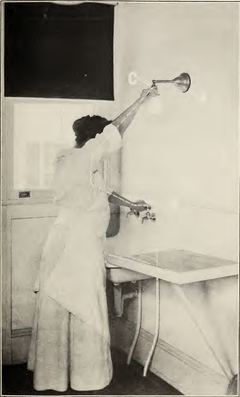
FIG. 8.—Illustration of the possible danger from shock by the passage of electricity from the metallic ungrounded fixture C (see insulating ring at base of fixture A), through the body to the grounded water faucet at B
