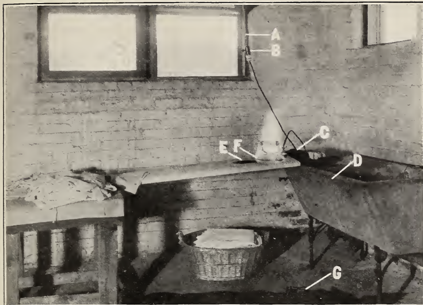
FIG. 6.—An improperly equipped and inadequately protected arrangement
