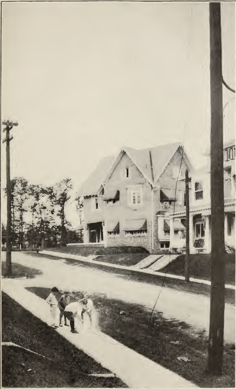
FIG. 4.— The fallen wire serves as an object of curiosity, especially where dangerous voltages cause flashing at the contacts with the earth
