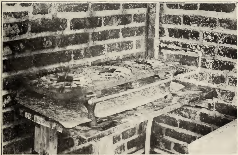
The same installation with defects corrected. The hot plate is connected with solid piping; the shelf has been covered with metal; a metal baffle has been placed between the burners and shelf top and the combustible materials have been removed
