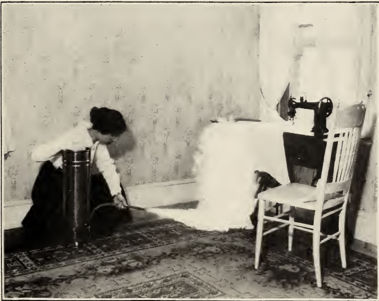
FIG. 25.—Soda-acid fire extinguisher, inverted at fire and set into action
