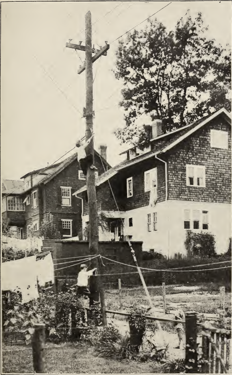
FIG. 3.— Illustration of possible danger to children climbing electric light poles
