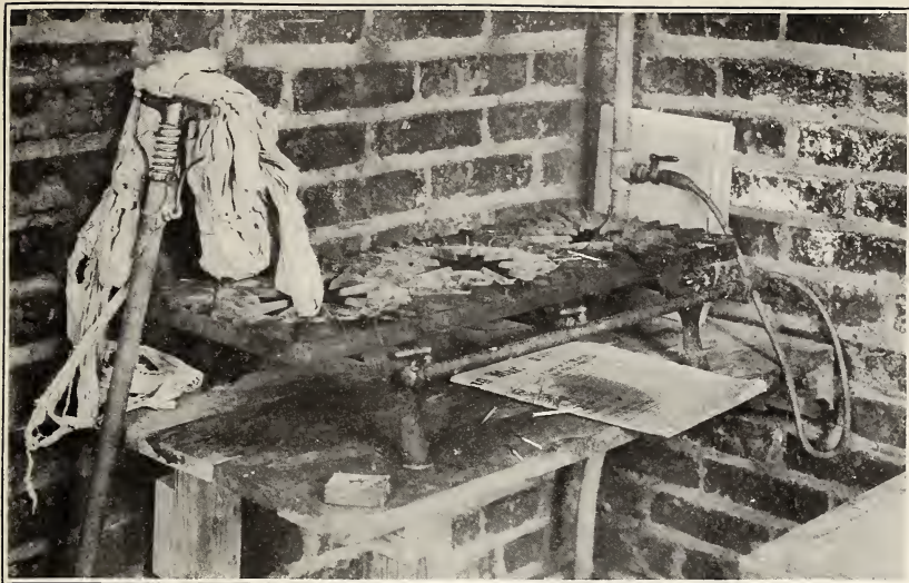
A poor installation; the hot plate is connected by flexible tubing with insecure ends of poor quality. Notice that gas supply is turned on at the pipe which would result in leakage if rubber ends split. The hot plate stands on a wood shelf with no protection between the burners and the shelf, which has been charred. Papers, matches, etc., are seen lying dangerously near to the burners
